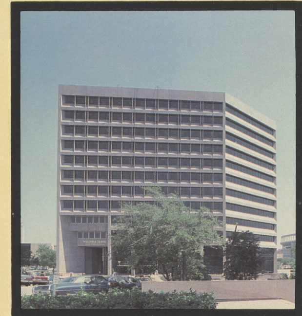
WILLIAM B. TRAVIS BUILDING
