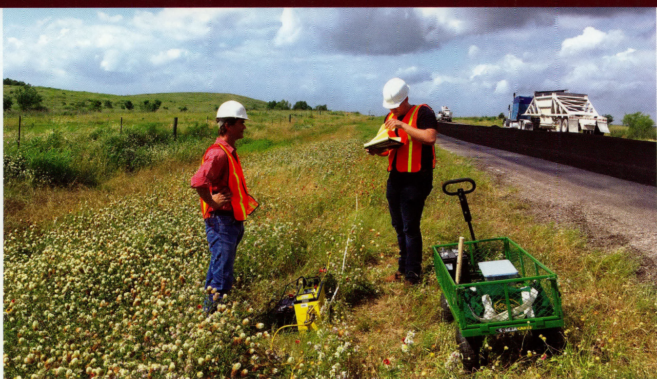
ERT highway maintenance project at FM-696 near Elgin, Texas.
