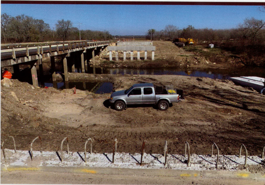
Above: ERT testing helped identify the best pier placements for new bridge construction near Yoakum, Texas.
