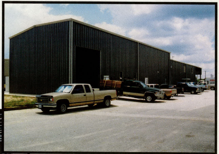
The new Maintenance Building includes a covered shipping and receiving area.
