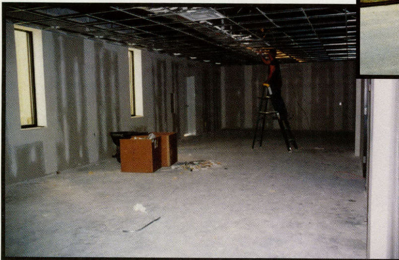
New lunch/meeting room during the final phases of construction.
