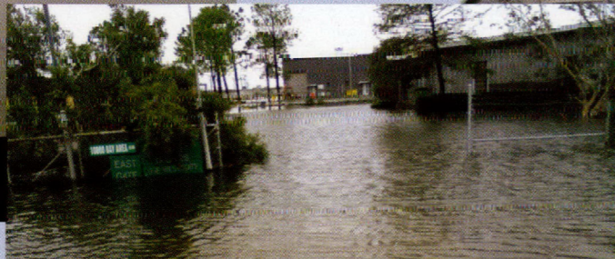
Entrance to Bayport and Central Lab.
