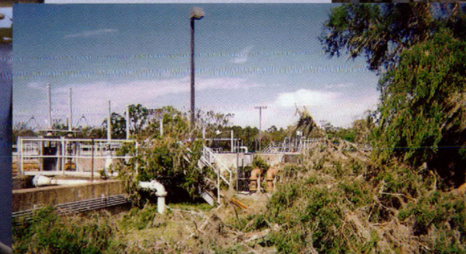
Trees at Blackhawk covering a portion of aeration basin.
