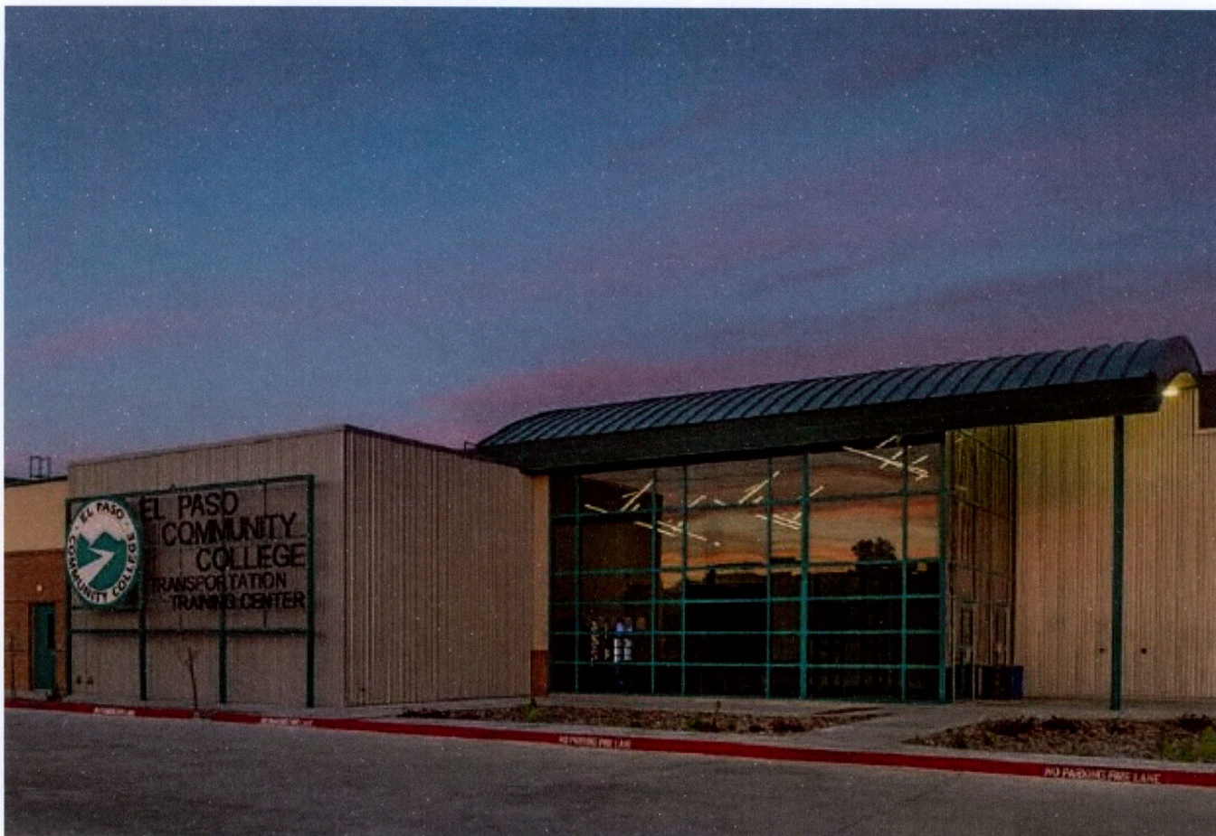
Transportation Training Center Valle Verde Campus
