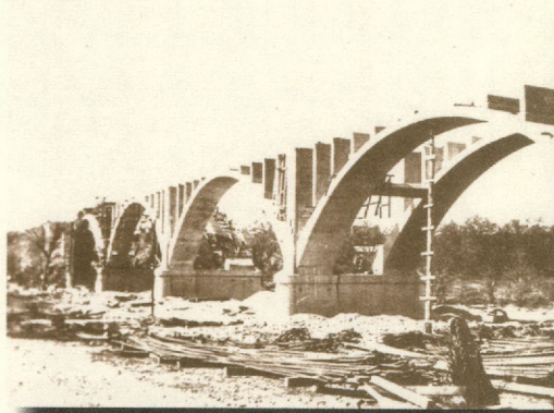
The Highway 81 Bridge at New Braunfels, Texas. Built in 1934, this concrete arch highway bridge now carries vehicular traffic along with parallel structures on adjacent IH-35. Photo courtesy of the Sophienburg Museum.
