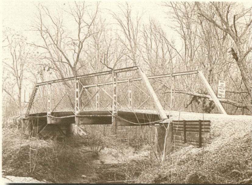
West Fork Bridge at Plum Creek in Caldwell County, Texas. Built by the Milwaukee Bridge & Iron Company, Milwaukee, Wisconsin in 1897, this 58 foot bridge is an excellent example of the pin-connected Pratt half-hip pony truss construction. Photo courtesy of the Caldwell County Genealogical Society.
