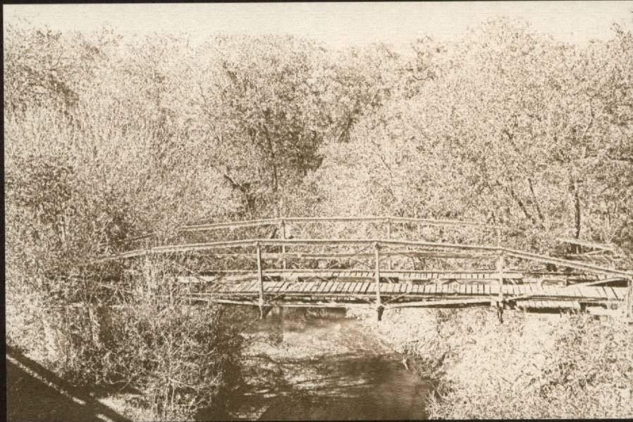
Soda Springs Bridge on County Road 130, Soda Springs, Texas. This 75-foot lenticular parabolic truss bridge was built in 1897 by the Berlin Bridge & Iron Company of New Berlin, Connecticut. It was closed to traffic in 1989 but was preserved for historic interest and can be viewed from the new bridge recently constructed next to it. Photo courtesy Caldwell Genealogical Society.
