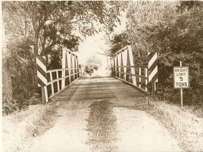
Bridge on County Road 173 near Lockhart, Texas. Built in 1895, this 90 foot lenticular parabolic truss bridge could only be built by the Berlin Bridge & Iron Company of New Berlin, Connecticut, since they held a patent for the design. Photo courtesy of Hays County Road and Bridge Department.
