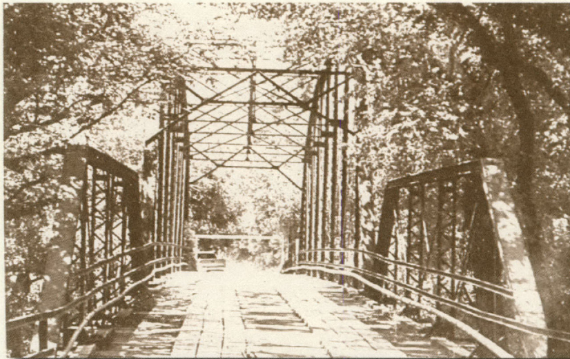
Guadalupe River Bridge at Oak Forest, Texas. This old steel truss bridge with wood planks served the community of Oak Forest, outside Gonzales, for many years. It was demolished and has been replaced with a newer structure. Photo courtesy of the Gonzales County Records Center and Archives.
