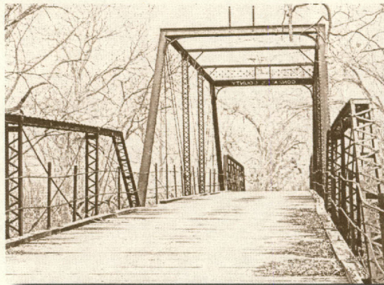
Slayden bridge over the San Marcos River in Gonzales County, Texas. This historic iron and wood deck bridge is still in use. Photo courtesy of the Gonzales County Records Center and Archives.
