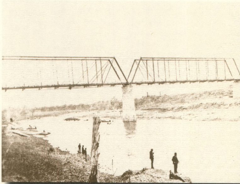
Faust Street Bridge at the Guadalupe River, New Braunfels, Texas. This unique bridge was built in 1887 by King Iron and Bridge Company of Cleveland, Ohio at a cost of $33,269. It is historically unique because of its wrought-iron construction and is the most complex and intact example of a large, multiple-span Whipple Truss roadway bridge surviving in Texas. When opened by Comal County, it was one of the first toll-free structures over a major waterway in Texas. Its 640 feet spans the Guadalupe River at a location that was originally a ford used by early settlers on the Old San Antonio Road (or Camino Real). It was the major crossing for traffic from Dallas-Austin-San Antonio from 1887 to 1934, when the state built a new bridge just downstream. In 1978, the Faust Street Bridge was closed to local traffic due to fire damage and is now reopened to carry pedestrians and bicyclists. Photo courtesy of the Sophienburg Museum.
