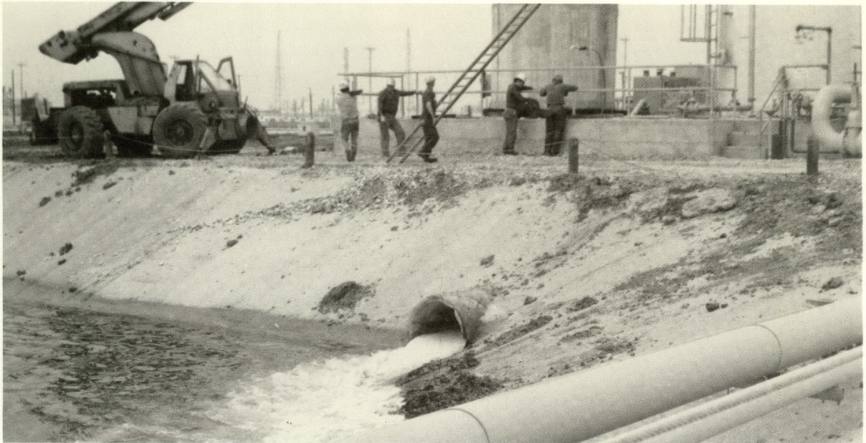
40 Acre receives first wastewater from Union Carbide. Final construction continues. 1974.
