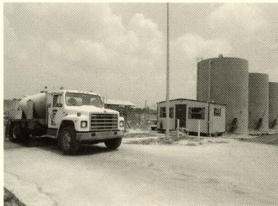
When the operators of portable toilet facilities in the Houston area needed a place to dispose of their waste, GCWDA was able in 1986 to provide the Vince Bayou Facility. Vacuum trucks discharge at Vince Bayou and wastes are sampled before being piped to the nearby Washburn Tunnel Facility for treatment.
