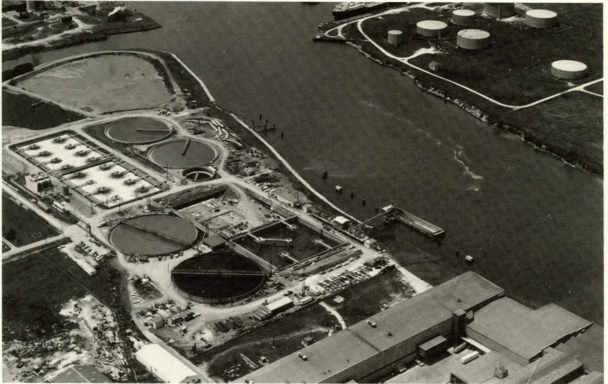
Washburn Tunnel Facility was referred to in a speech by Gov. Dolph Briscoe as a "unique experiment" that symbolizes the rebirth of the Houston Ship Channel. (1976)
