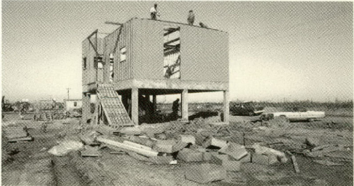
Campbell Bayou construction.
