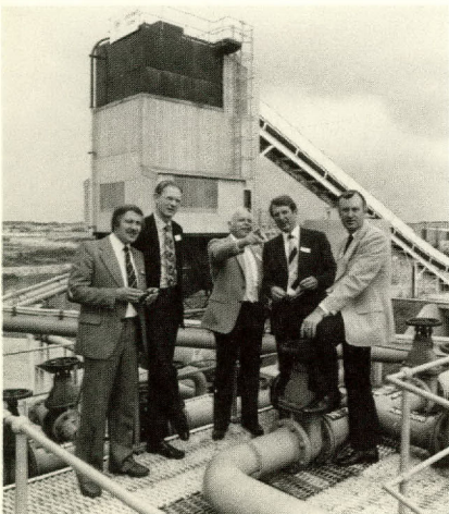
Stablex Facility, London.
