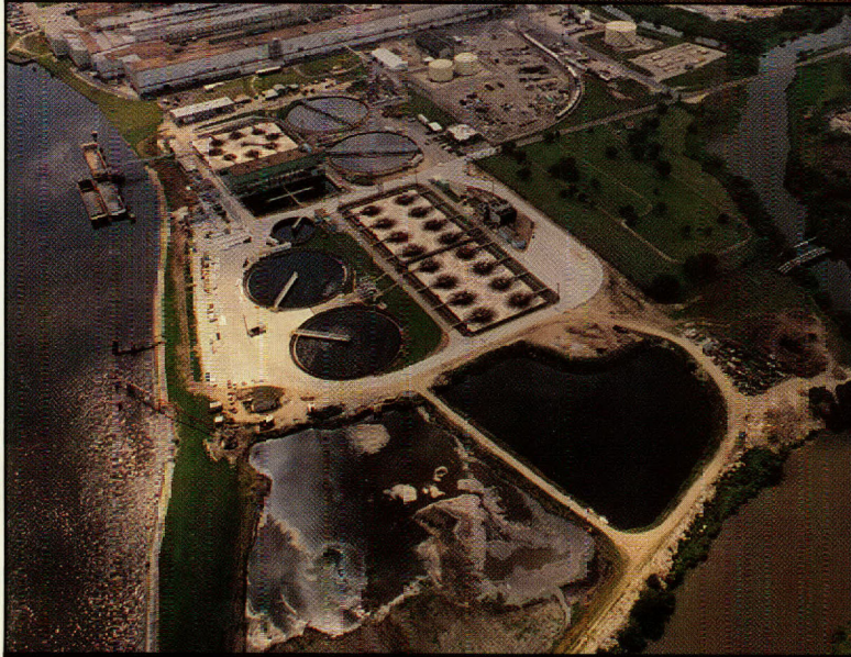
The Authority's Washburn Tunnel Facility provides a clear example of how GCA provides cost efficient services to industry by treating its wastewater to acceptable environmental standards. Nearly a dozen industrial plants send millions of gallons of wastewater through this facility daily. The co-mingling of waste streams is effective for balancing pH values and for a number of other applications.
