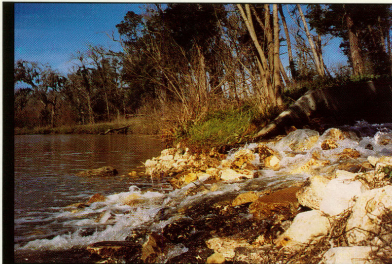
Clean, thoroughly treated water—our finished product—leaves the Blackhawk Facility's discharge flume from where it flows directly into Clear Creek.
