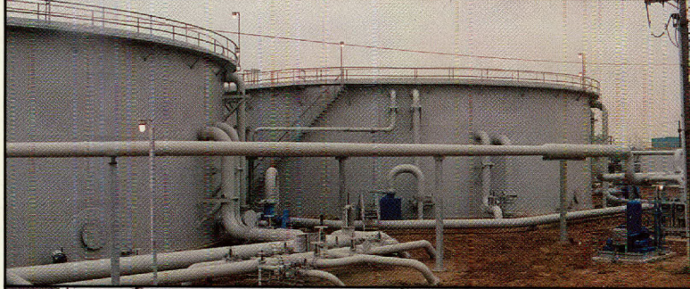
Bayport's first stage treatment system was upgraded with the addition of two aboveground treatment tanks that replaced a shallow aerated basin.
