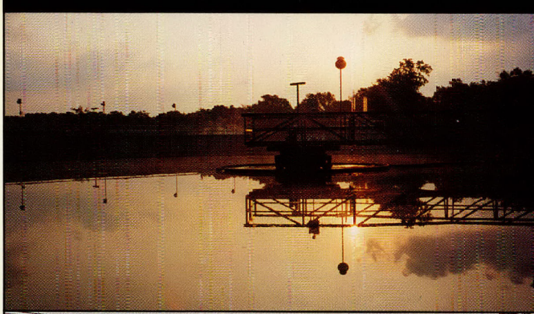
Night quickens over the Blackhawk Facility, GCA's premiere municipal wastewater treatment plant located in Friendswood.
