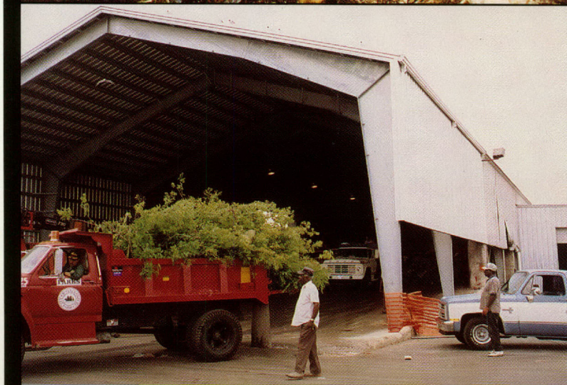
Added roof area at Galveston's Transfer Station Facility expedites garbage transfer processing from municipal trucks to GCA transports.
