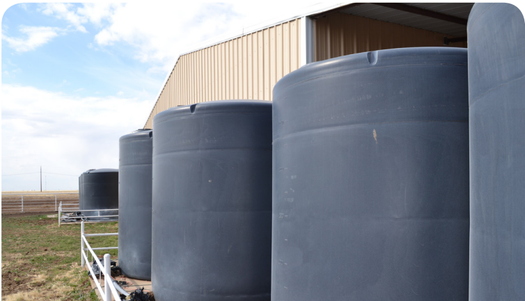
Each tank holds 3,000 gallons of rainwater.
