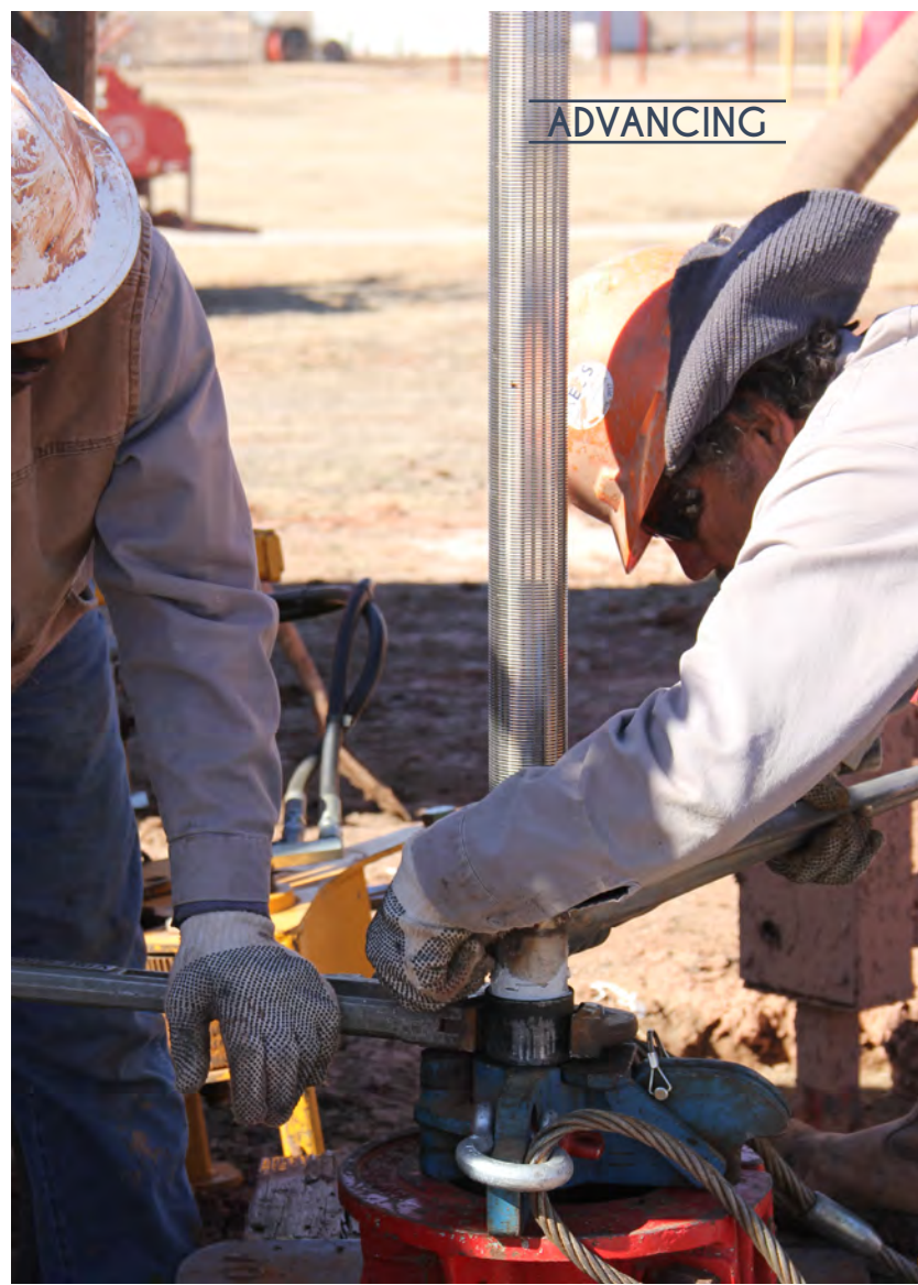
Installing screen in Dockum Aquifer test well at Abernathy
