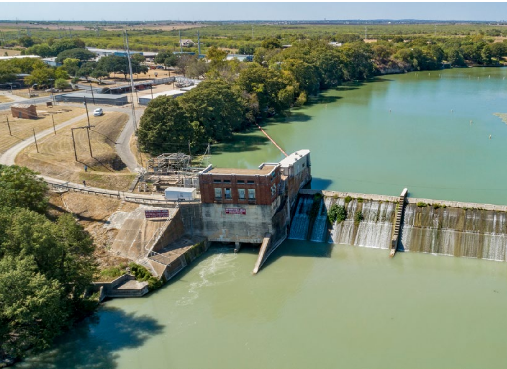
Aerial view of Lake McQueeney Dam.
