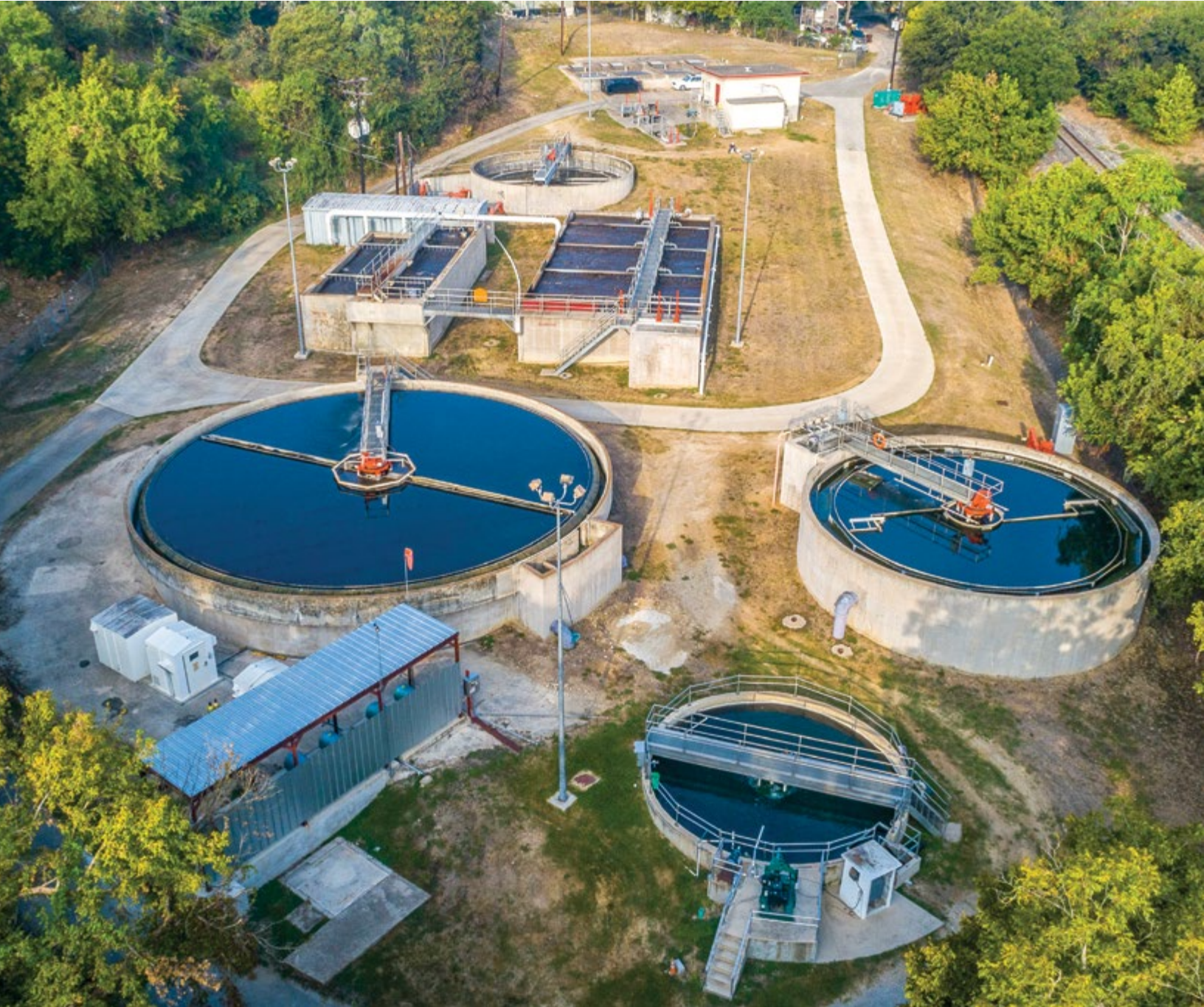
The Larremore Wastewater Treatment Plant can treat up to 1.1 million gallons of wastewater per day, and serves the city of Lockhart, TX.
