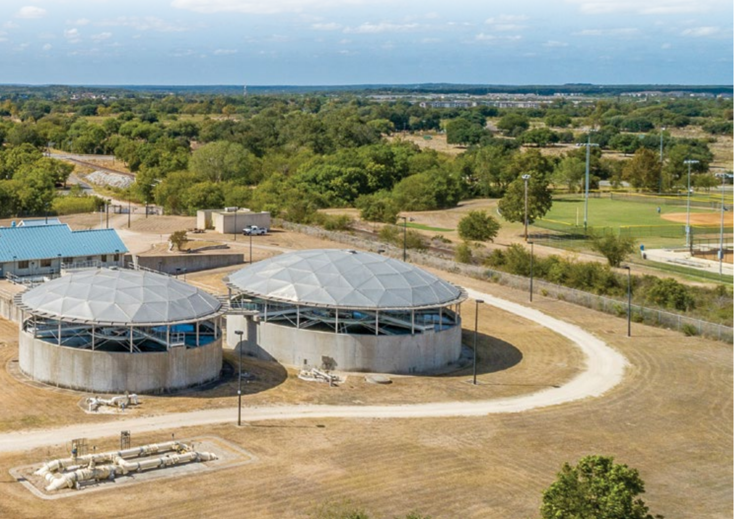
Aerial view of the San Marcos Water Treatment Plant.
