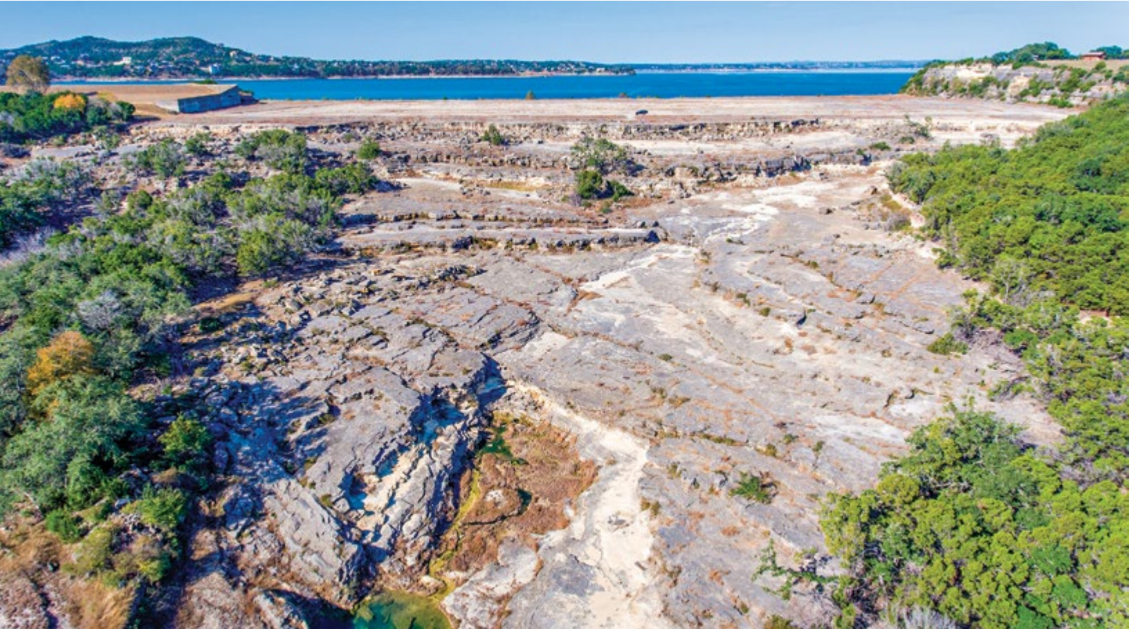
View of the Canyon Lake Dam spillway from the Gorge.
