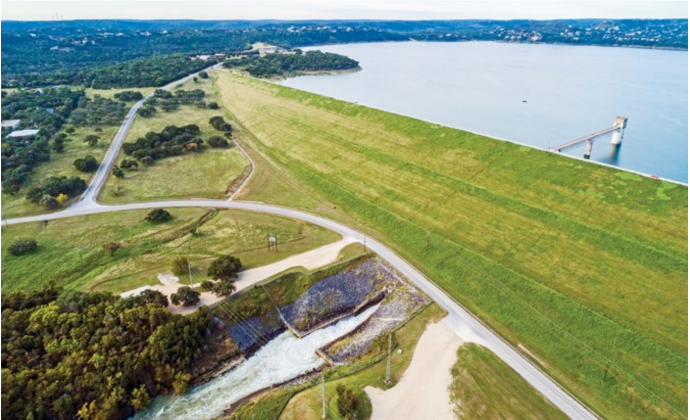
Water is released from Canyon Reservoir through a U.S. Army Corps of Engineers conduit.
