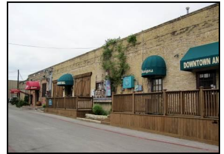
Businesses in this cleaned-up alley in New Braunfels utilize their back doors as secondary entrances.
