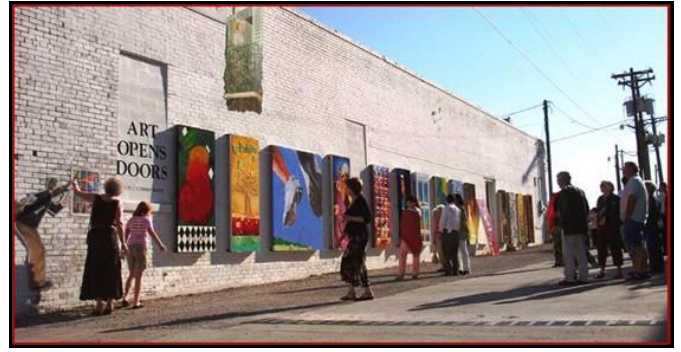
The Art Opens Doors alley project in downtown San Angelo affixes artwork to the mortar rather than the masonry.
