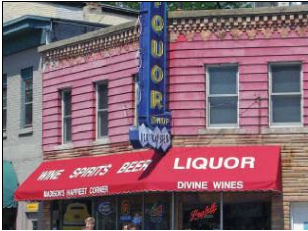
This faded aluminum siding is obviously concealing an original brick wall.
