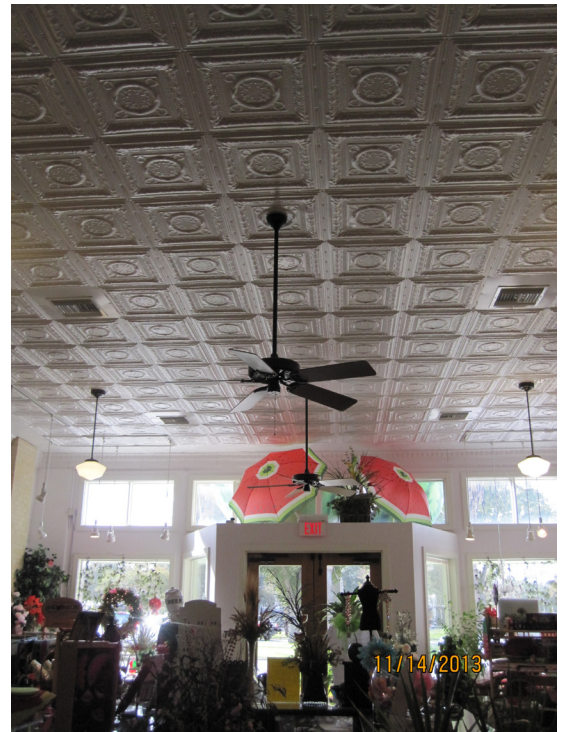
Pressed tin ceiling in historic building in Luling.
