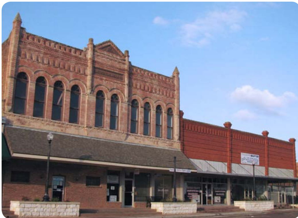
In the early 2010s, the city completed a renovation of the sidewalks and historic style lamps in portions of downtown.
