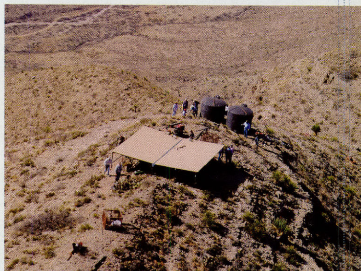
Volunteers with the Texas Bighorn Society install a rainwater collection system that will fill a wildlife "guzzler" in the Baylor Mountains near Van Horn last spring. The guzzler's automatically refilling trough provides much-needed drinking water for all types of wildlife in remote areas like this.
