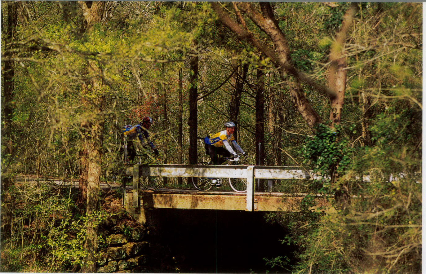
CCC crews of the 1930s built Park Road 1-C to connect the two state parks. Loblolly pines grow thick along the route, providing a canopy of shade for cyclists at several points.
