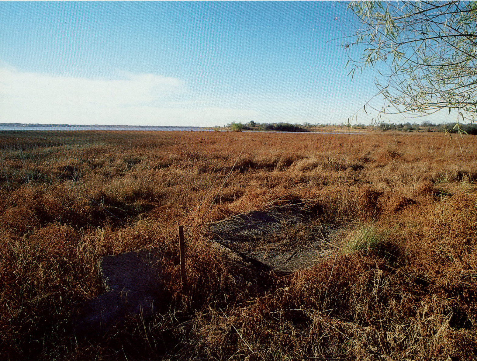
Broken cement foundation slabs are all that remain of the old town of Hagerman. Most folks had left by 1943 when rising waters from Lake Texoma started lapping at the town's outskirts.
