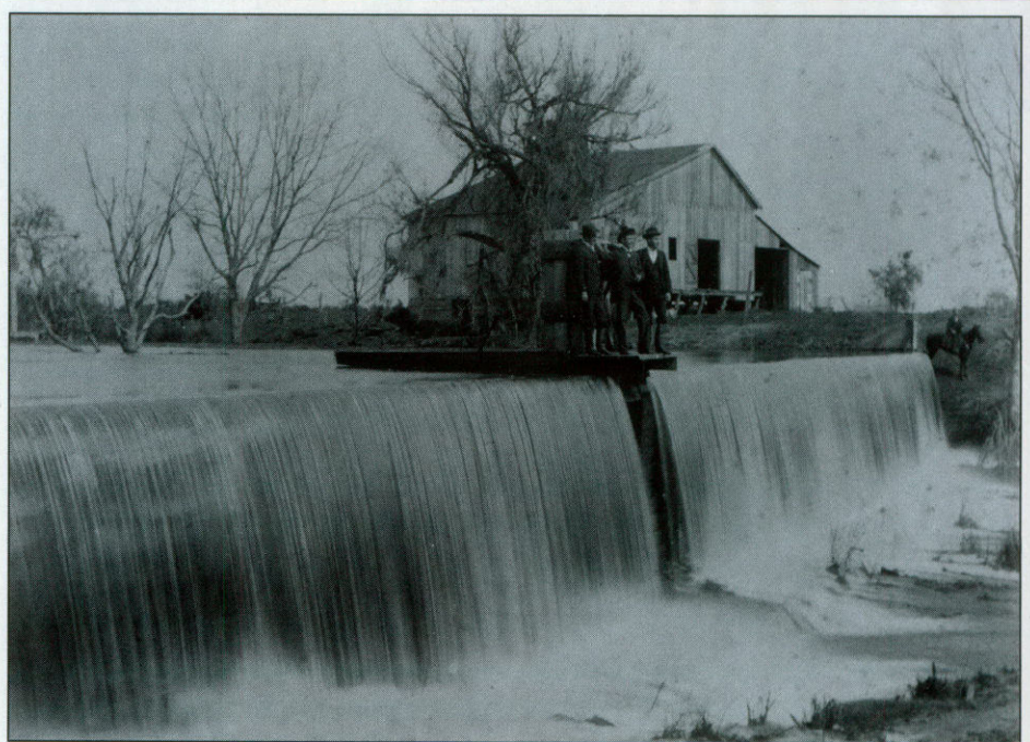
The San Marcos River circa 1893 in the Martindale area. Some four miles from the headwaters the Blanco River flows into the San Marcos, causing the San Marcos to become a more typical Central Texas stream. Dams were built in the San Marcos, Martindale and Staples areas to create water power.
