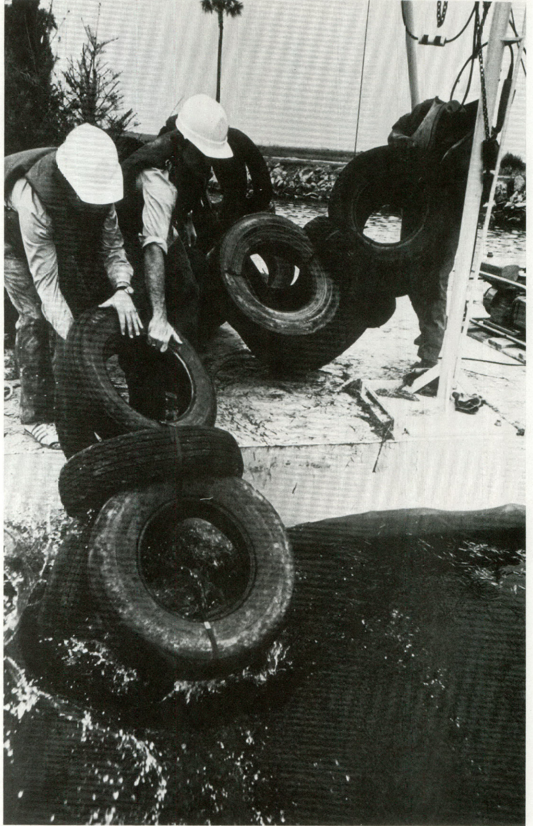
A special barge has been constructed to build and sink fish attractors in Texas lakes. It can handle large numbers of tires, cedar trees, stakes and other reef-building material.
