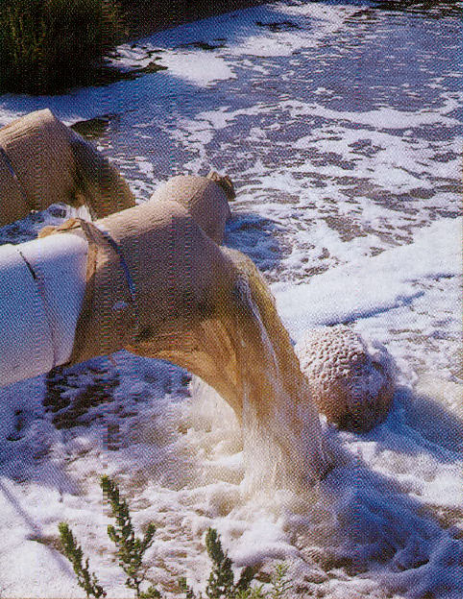
Bags filter incoming water to Loma Alta Aquaculture. Much of the water is recirculated and purified through wetlands.
