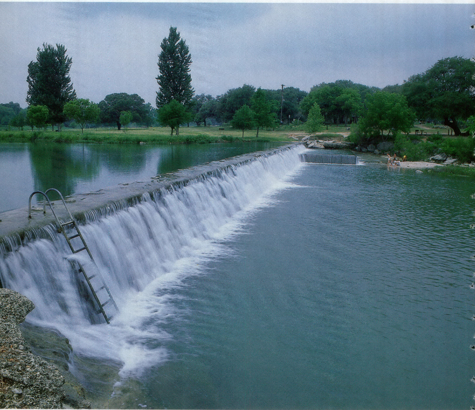
In the 1930s, Civilian Conservation Corps workers used quarried limestone to build two dams across the river. CCC workers also built the park's picnic tables and an arched bridge.
