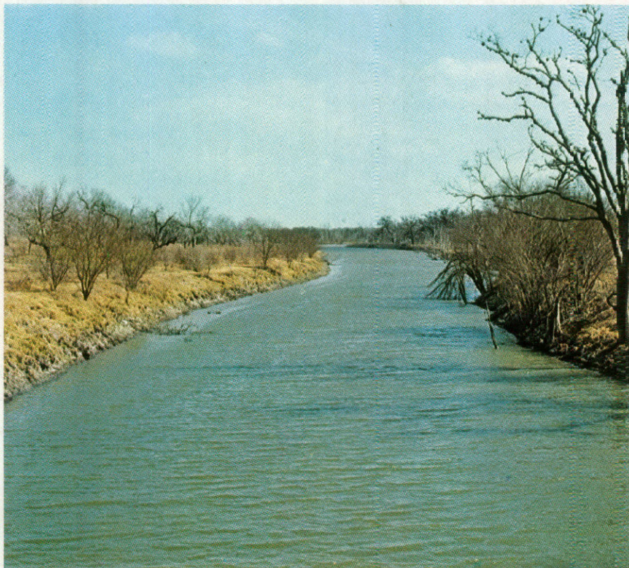
Clearing a waterway that is completely choked with water hyacinths makes it available for irrigation purposes, flood control, water storage and recreation.
