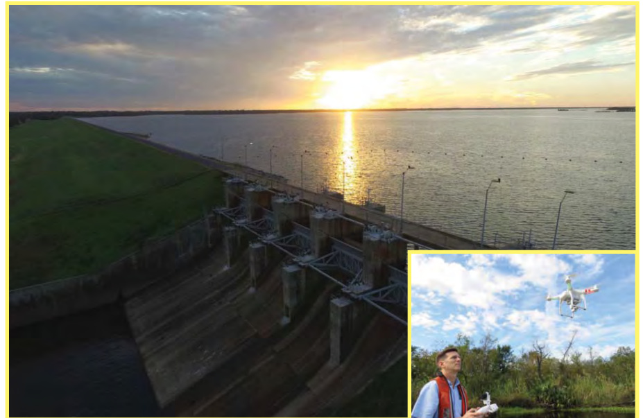
Aerial Drone Photography, Lake Fork Reservoir and Dam
