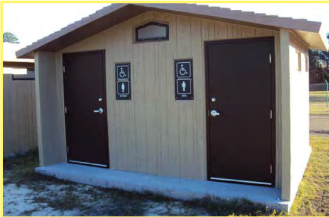
Precast Concrete Vault Toilet Building
