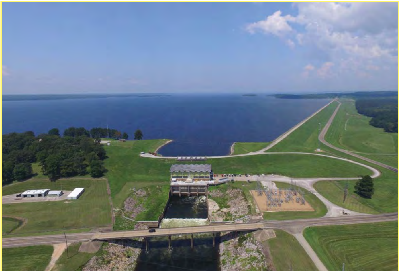
Toledo Bend Dam and Powerhouse
