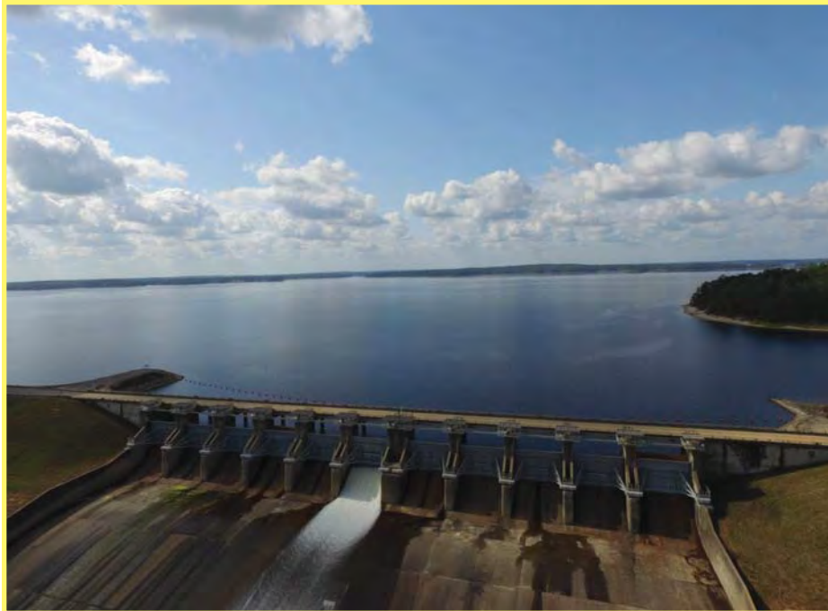
Toledo Bend Spillway Gate Refurbishment Project Completed
