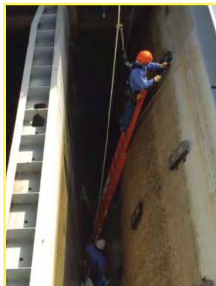
Tainter Gate Cathodic Protection Maintenance
