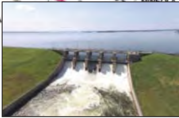
Lake Fork Dam & Reservoir
