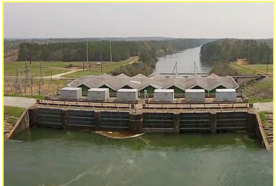
Powerhouse Intake and Trash Racks
