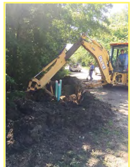
Wastewater Line Repairs
