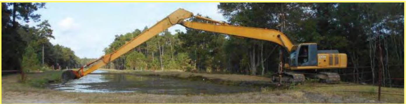
Mechanical Removal of Vegetation from the Water Supply Canal
