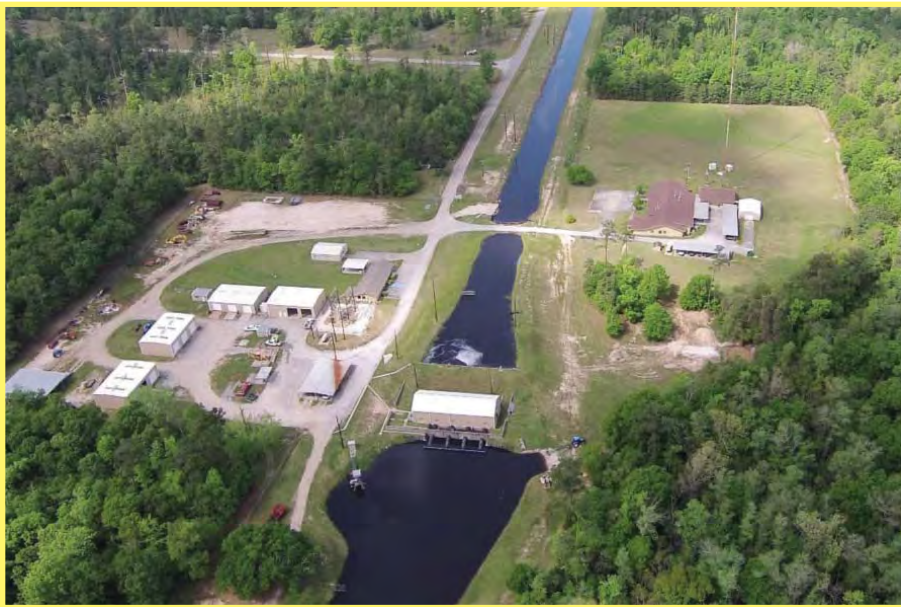
Gulf Coast Division Pumping Plant and Canal
