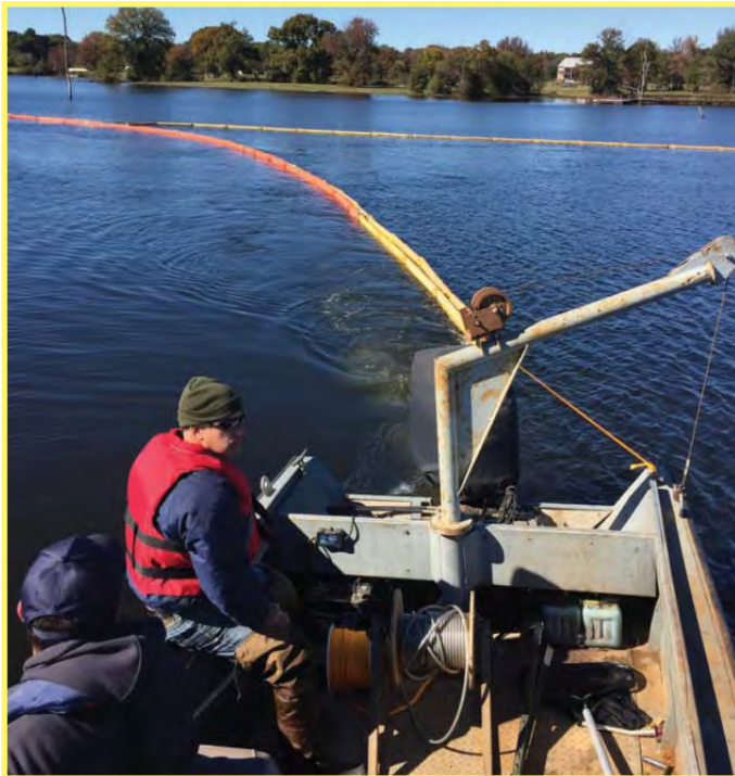
Deployment of Booms to Control Giant Salvinia
