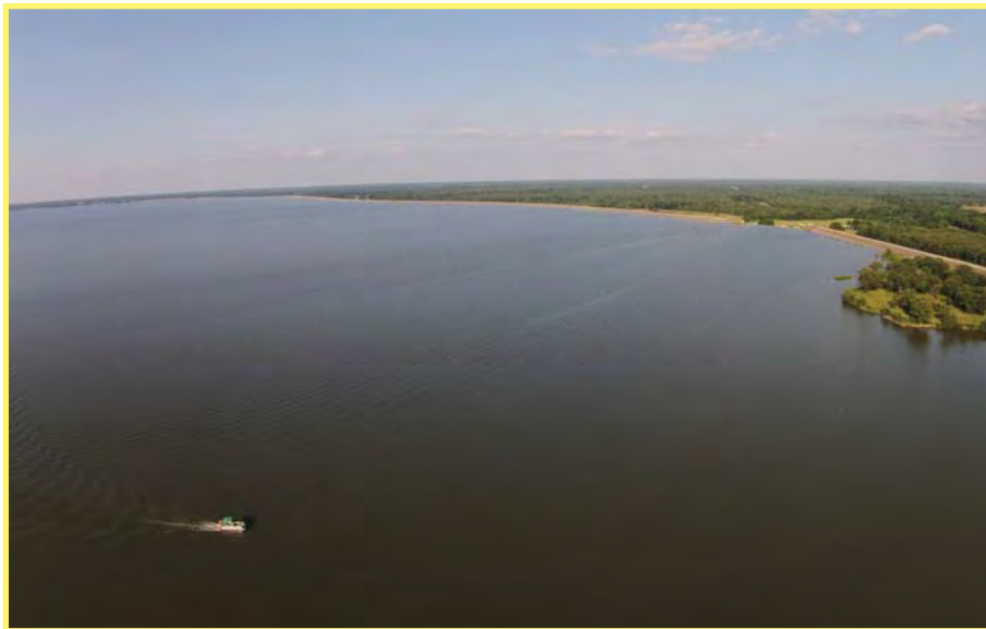
Iron Bridge Dam and Reservoir
