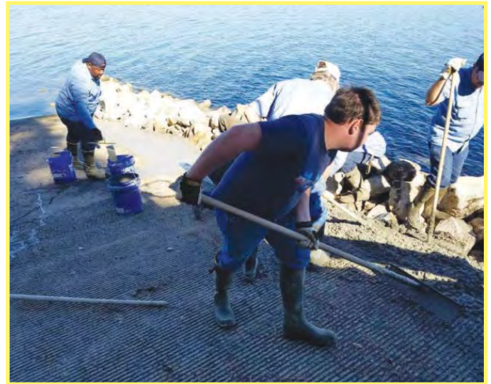
East Hamilton Boat Ramp Repairs
