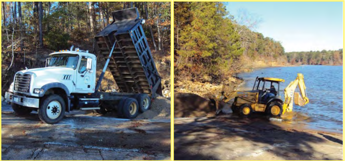
East Hamilton Boat Ramp Maintenance and Repair
