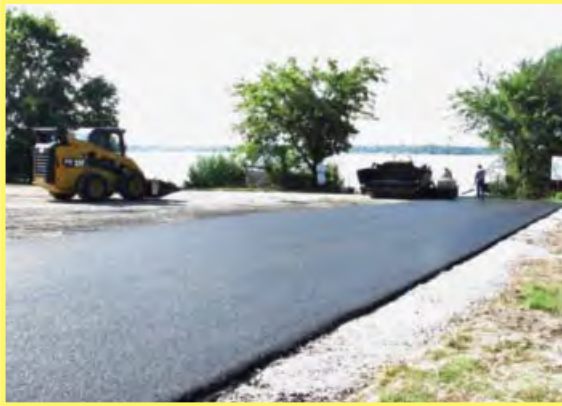
Improvements to the Caddo Boat Ramp Parking Area
