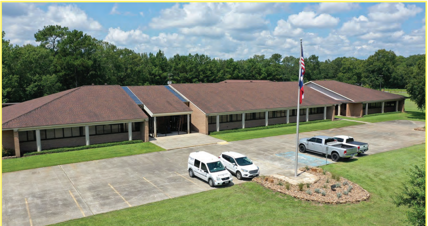
Sabine River Authority General Office
