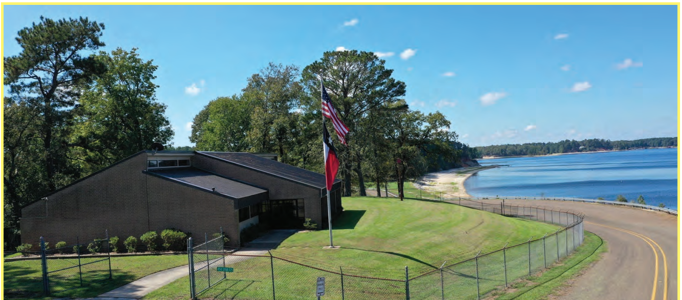
SRA, Toledo Bend Division Offices
