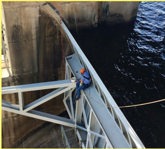
Tainter Gate Maintenance
