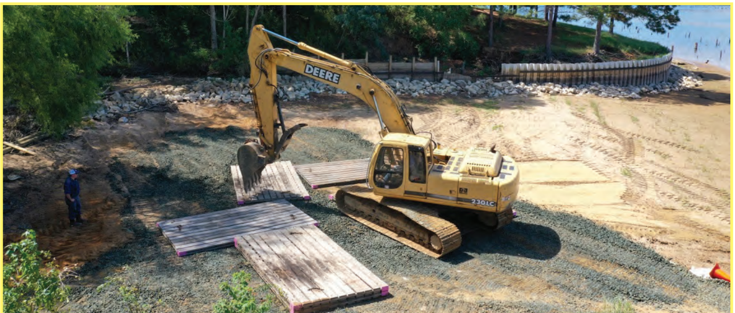
Taking Advantage of Low Water Levels for Shoreline Stabilization Work
