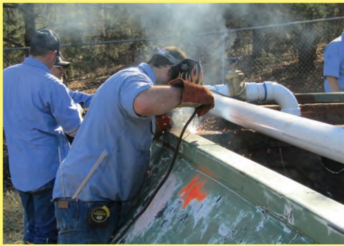
Repairs to Waste Water Treatment Facility
