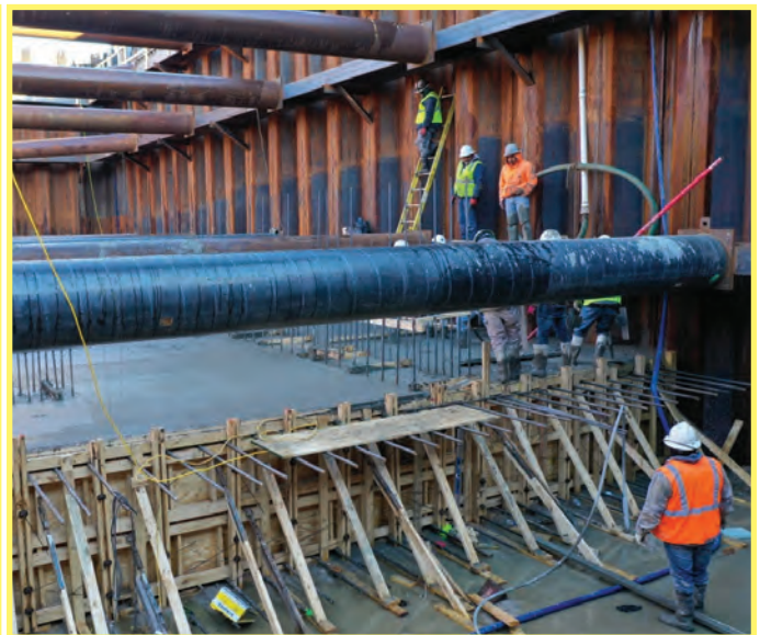
Pump Station Wet Well with Center Section Floor Being Finished
