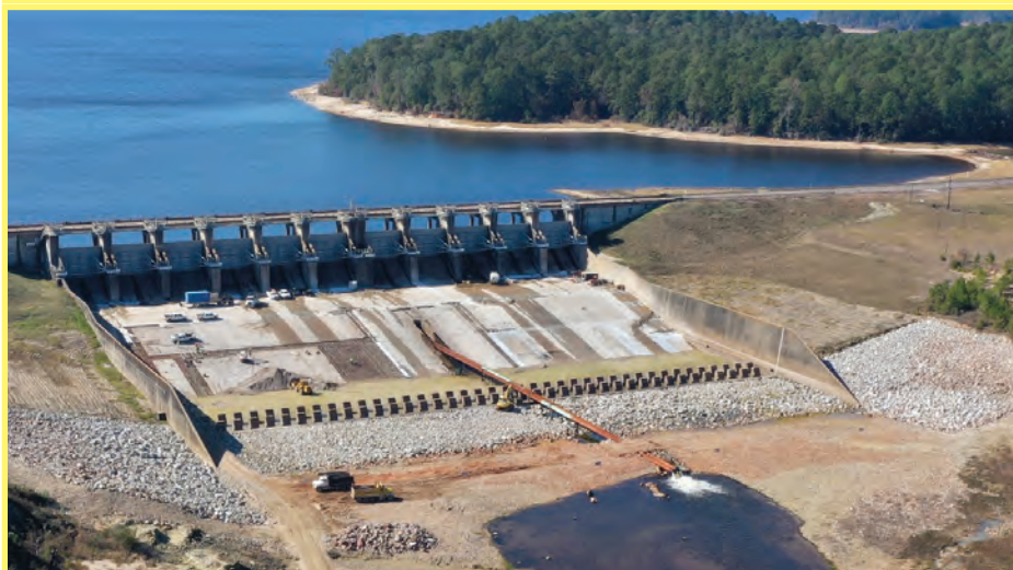
December 2018 (top) and November 2019 (bottom) Spillway Repairs
