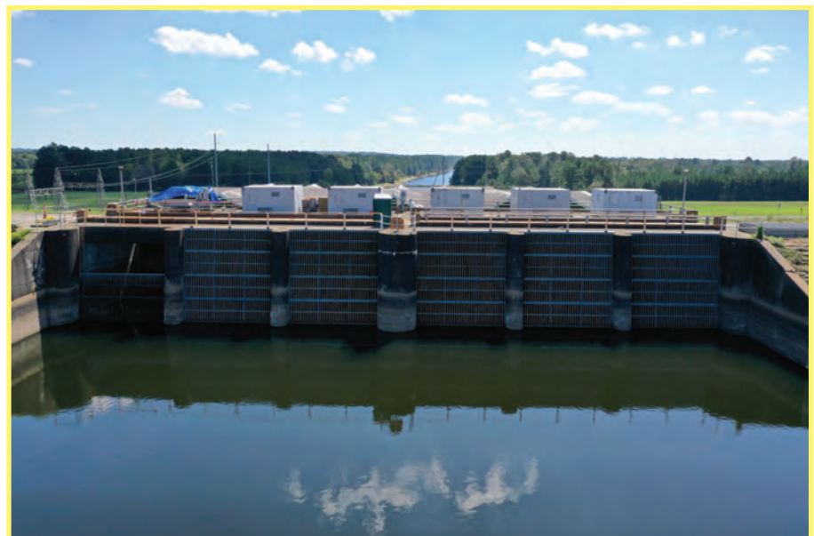
Toledo Bend Powerhouse, New Forebay Trash Racks
