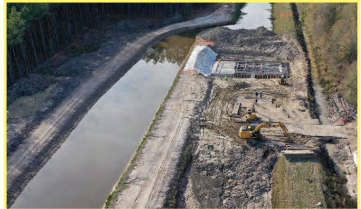
Construction of canal bypass and new pipeline termination structure
