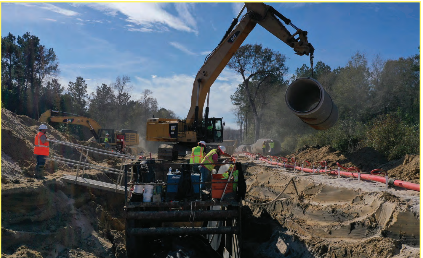
Laying 66-inch Pipe in the 7-Mile Right-of-Way
