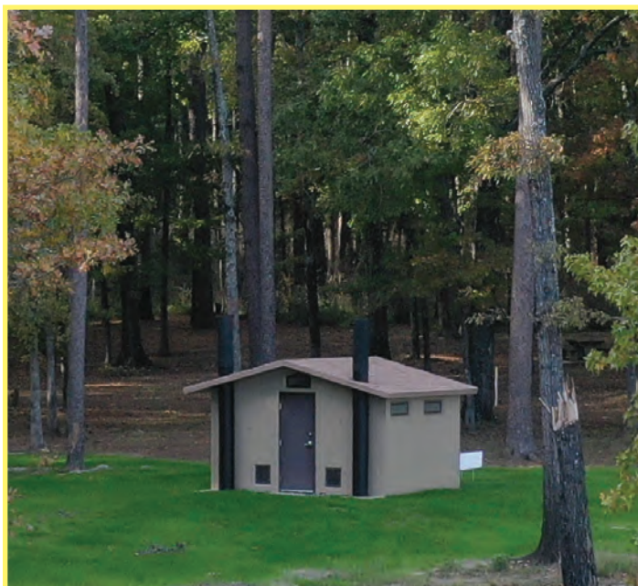
New Restroom Facility at the Lakeview Recreation Site
