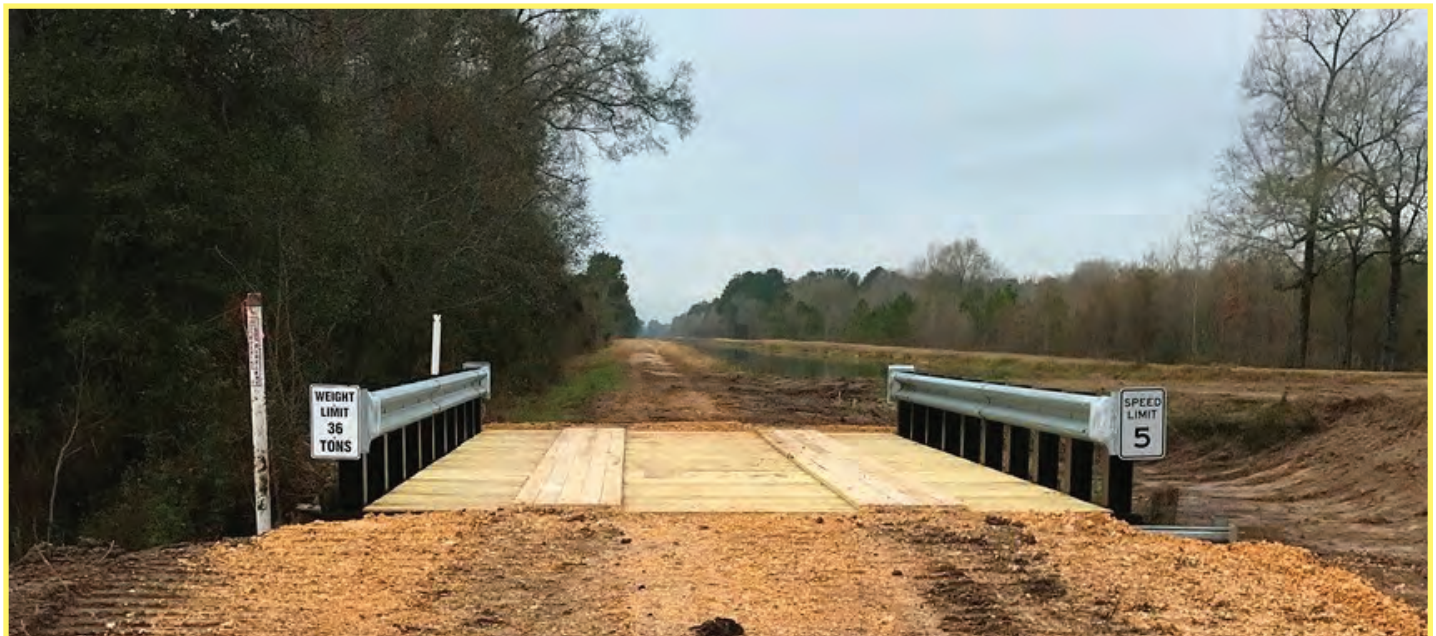
New canal right-of-way bridge spanning an Orange County drainage ditch
