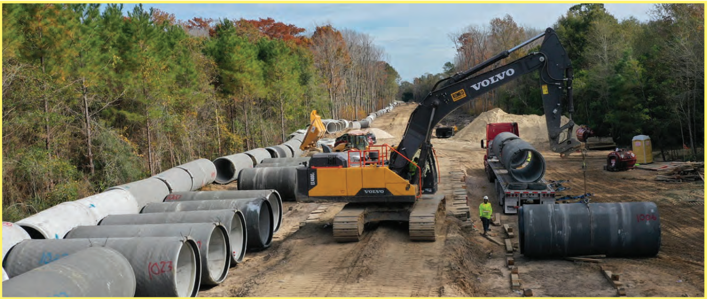
Offloading Concrete Pipe Into the Cleared Right-of-Way
