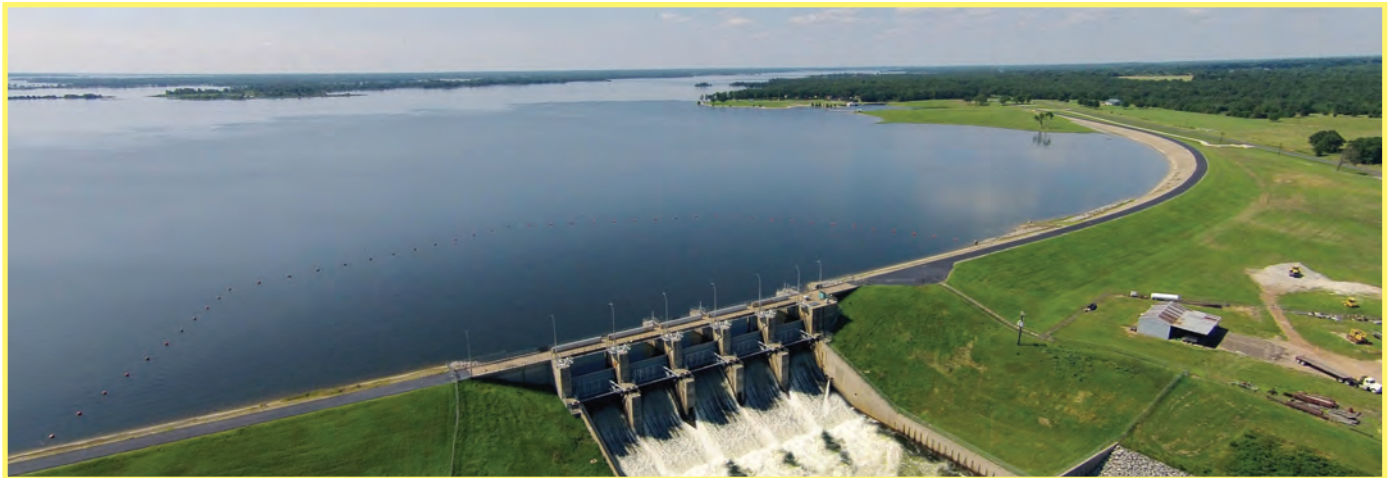
Lake Fork Dam and Reservoir
