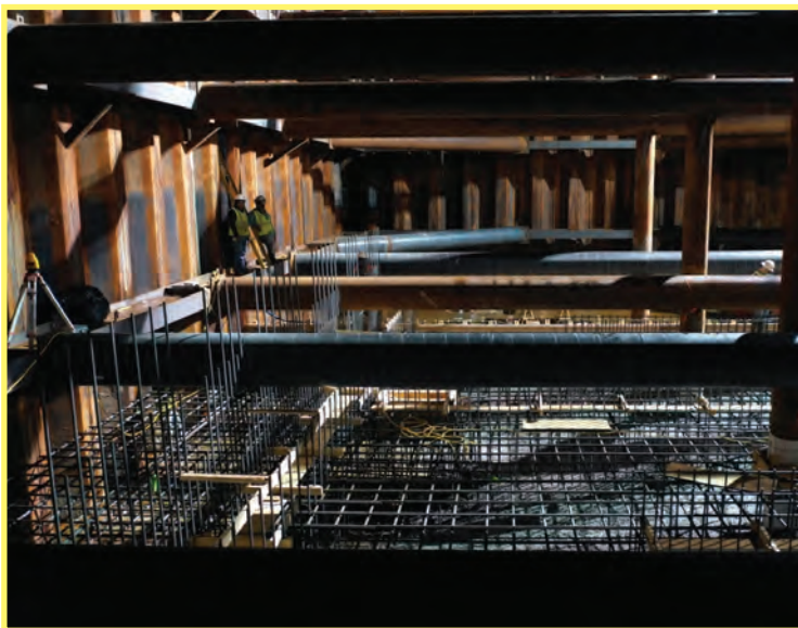
Pump Station Wet Well Steel Reinforcement Prior to Concrete Placement
