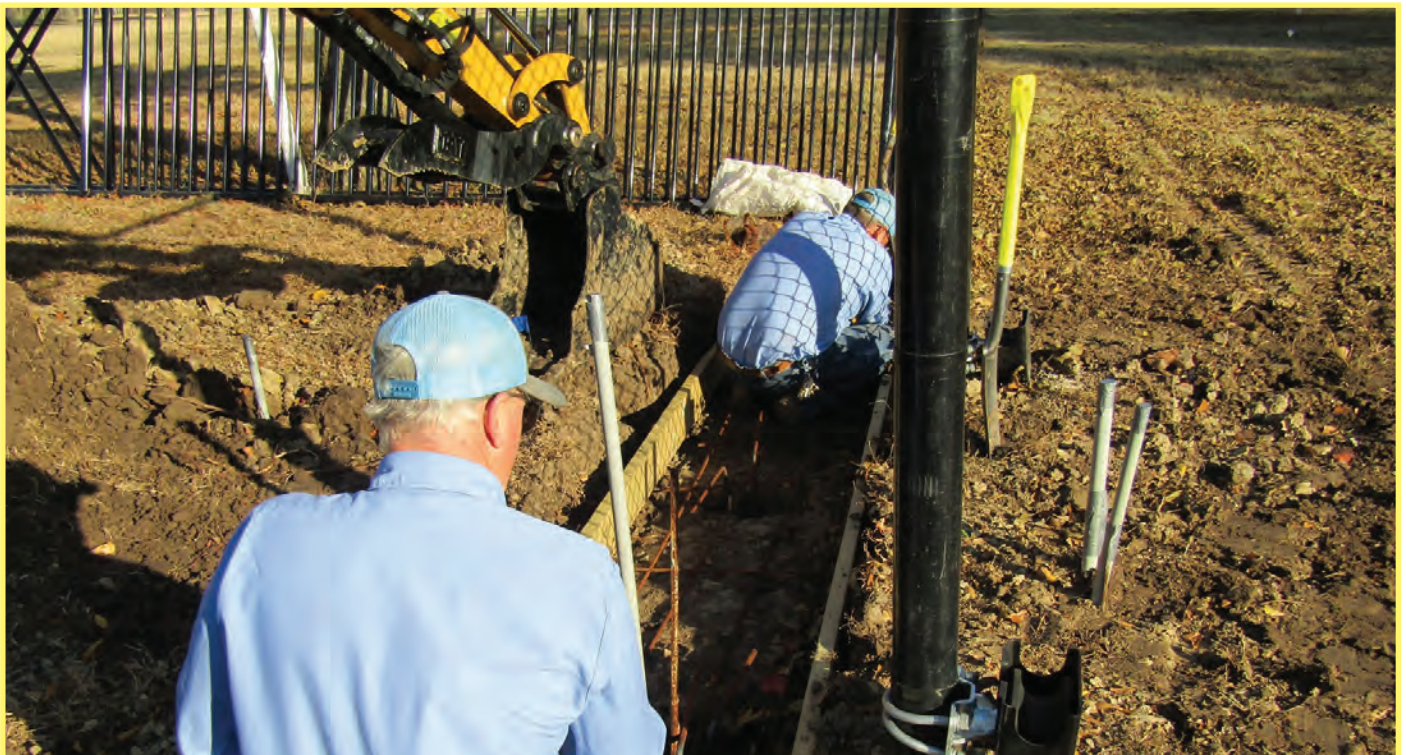
Lake Tawakoni Division Offices Entry Gate Upgrade
