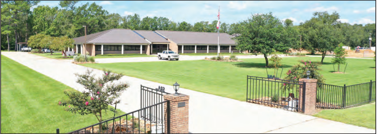
Sabine River Authority General Office
