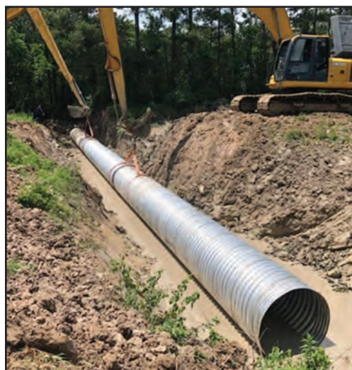
FM 1442 Underdrain Project
