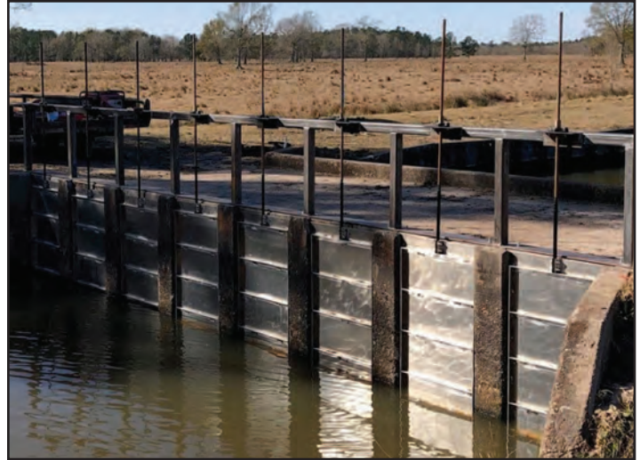
8-Gate Refurbishment Project
