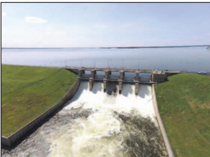
Lake Fork Dam and Reservoir
