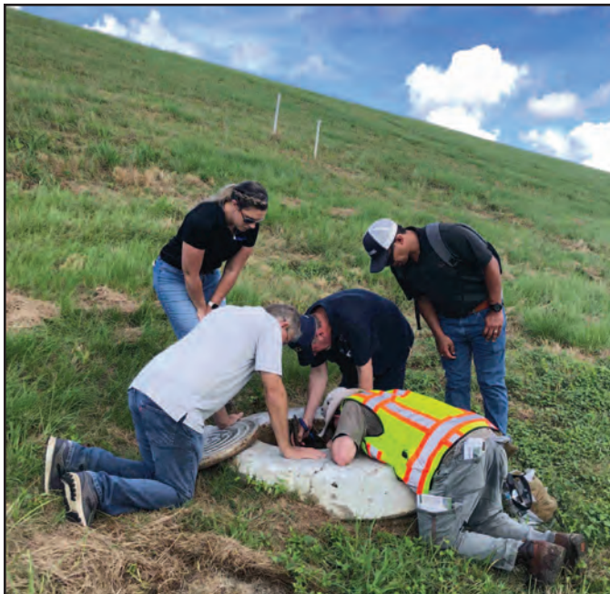
FERC Inspection of the Underdrain System
