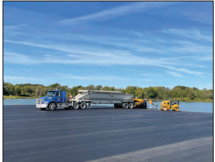
Paved Parking at Lake Tawakoni Recreation Site
