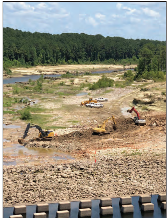
Removing Coffer Dam on Spillway Channel
