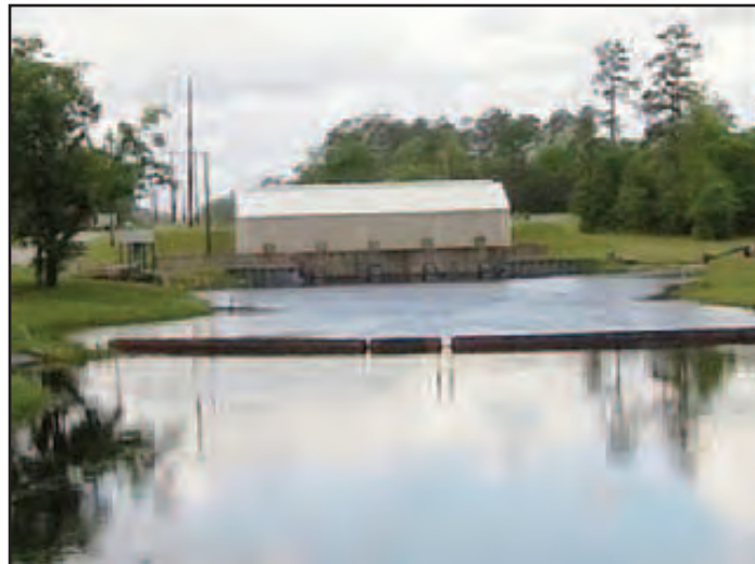
John W. Simmons Gulf Coast Canal Pump Station
