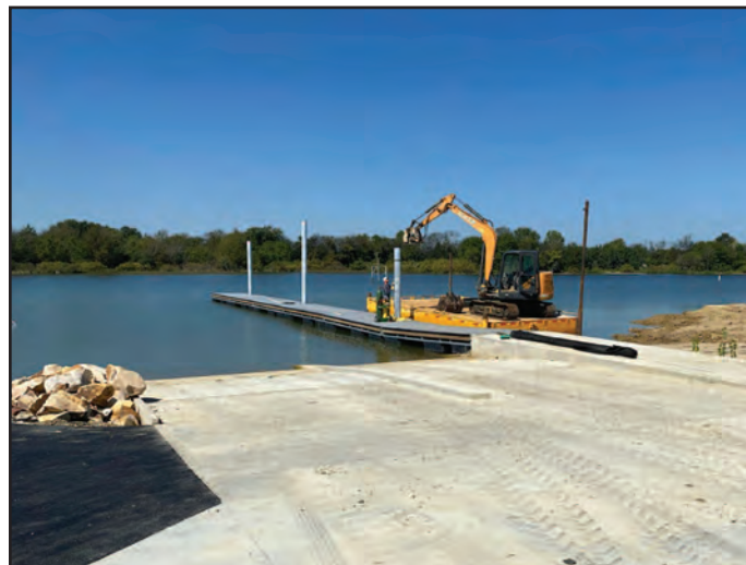
Floating Pier Construction
