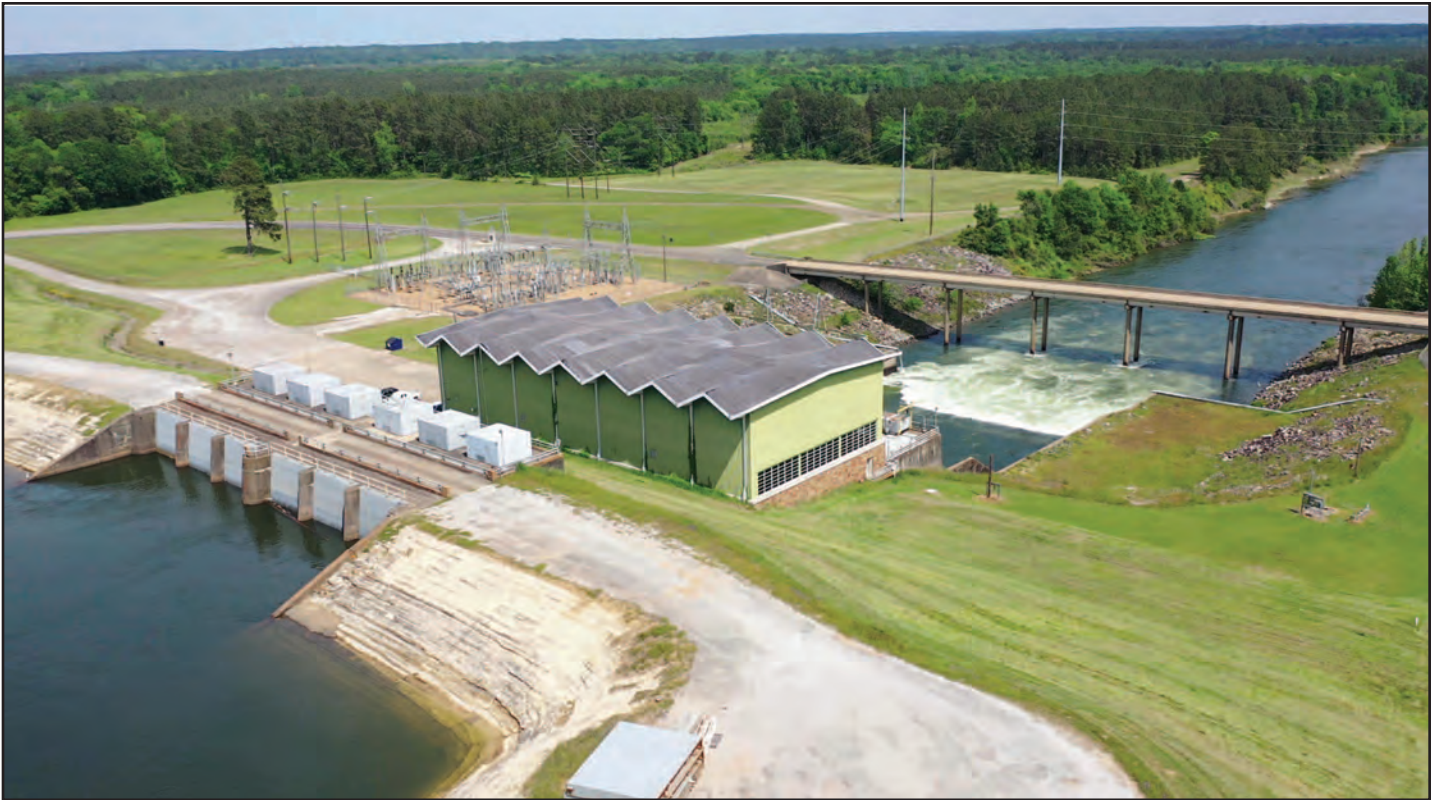
Toledo Bend Powerhouse
