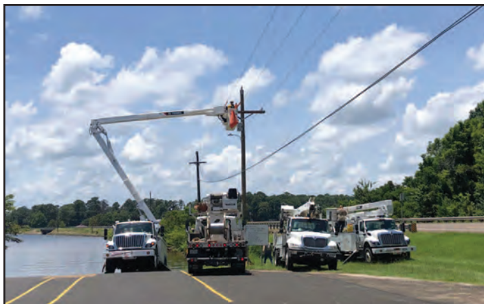
Installation of Security Light at Carrice Creek Boat Ramp
