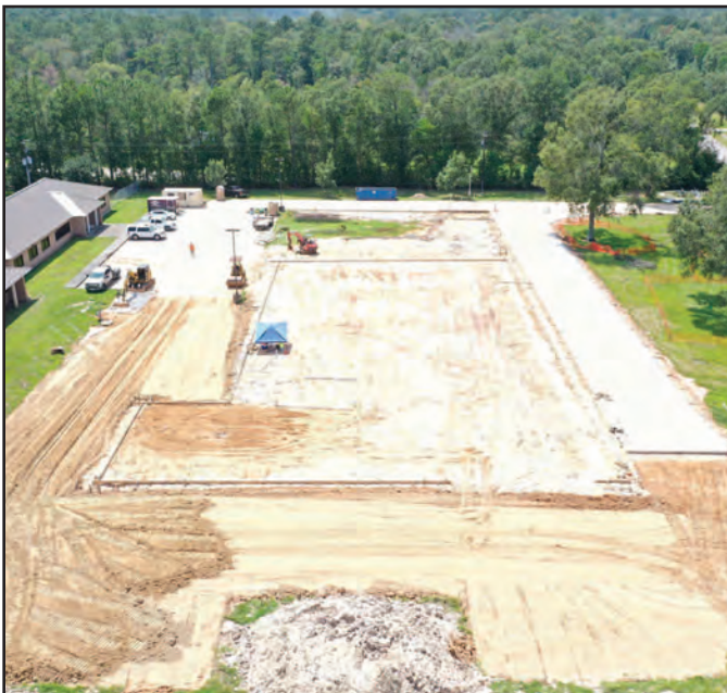
Initial Site Preparation for the New ESD Building
