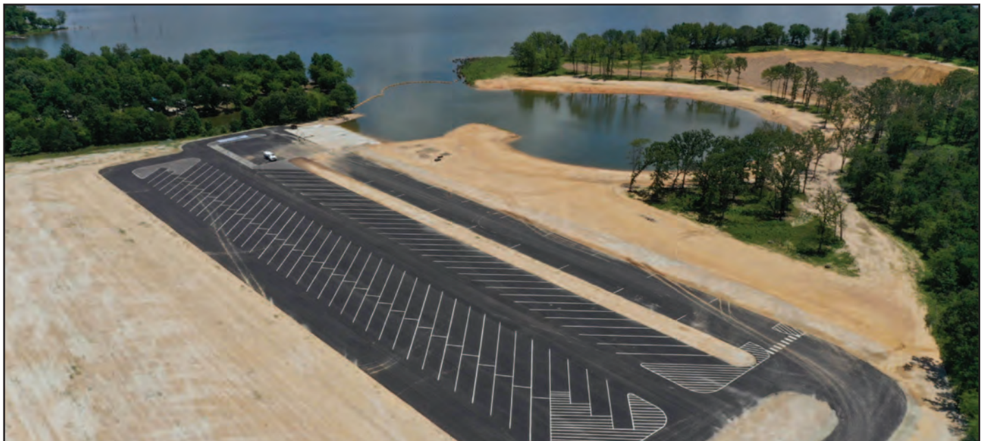
Parking Lot and Six-Lane Boat Ramp at Caney Point Recreation Area
