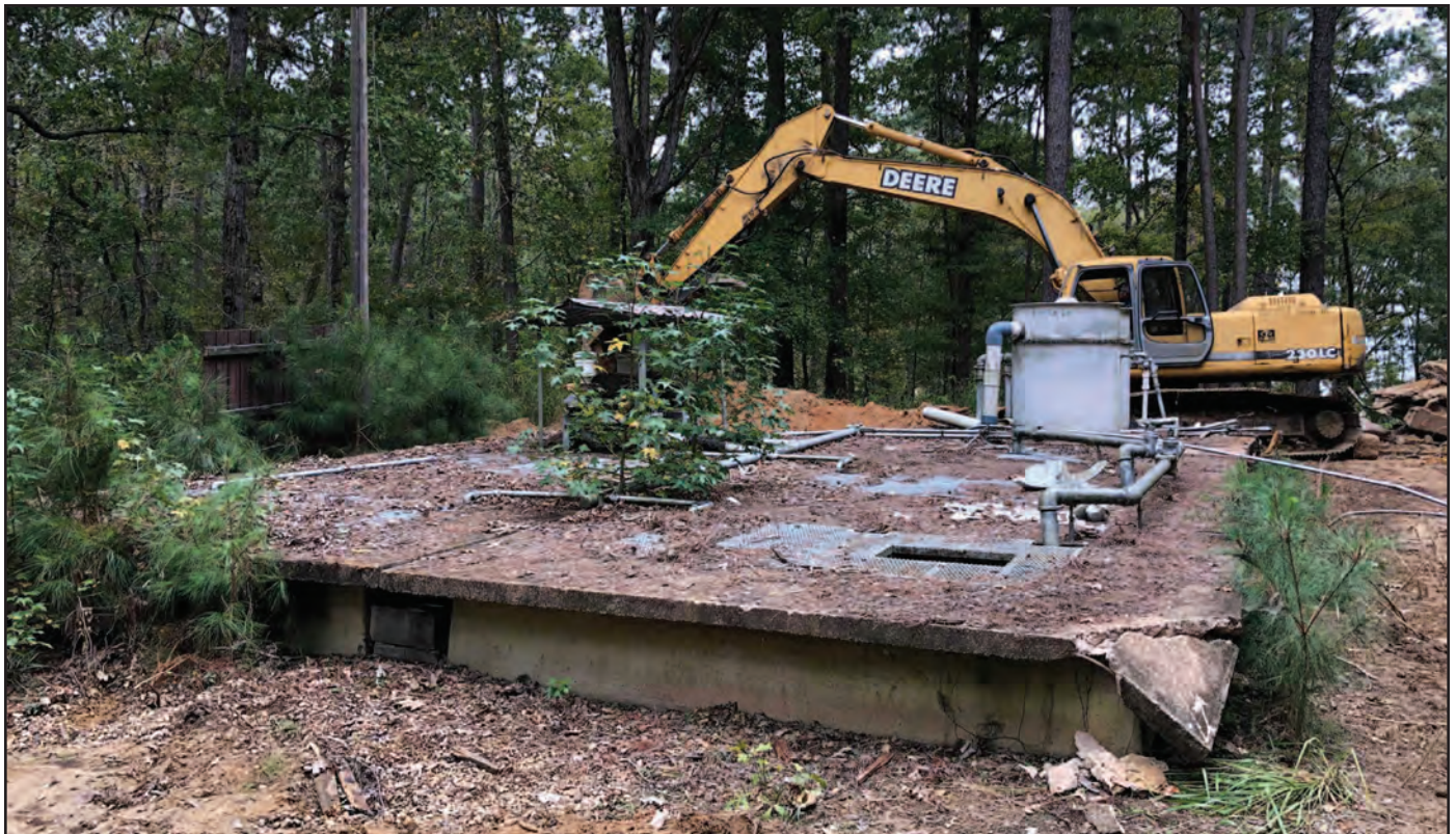
Demolition of Wastewater Treatment Facility at Ragtown
