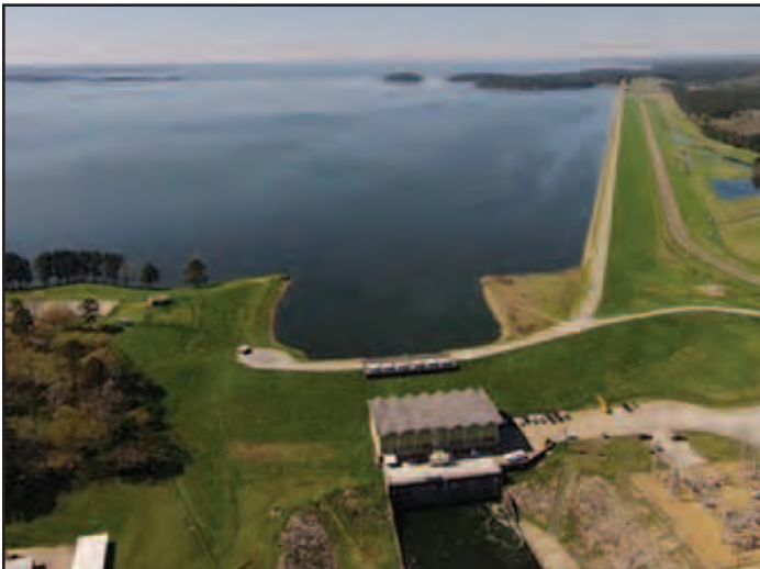
Toledo Bend Dam and Reservoir
