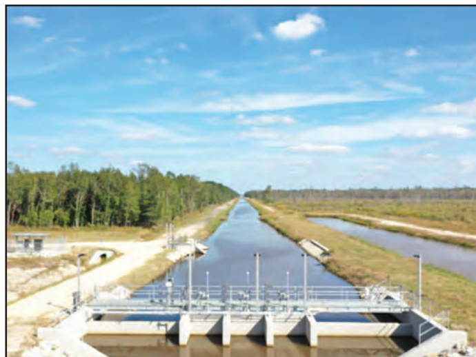
Canal Connection Slide Gates
