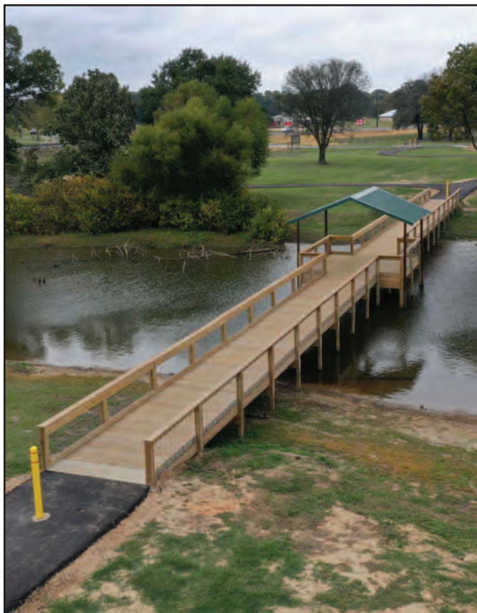
Footbridge Over Cove at Swearingen Park
