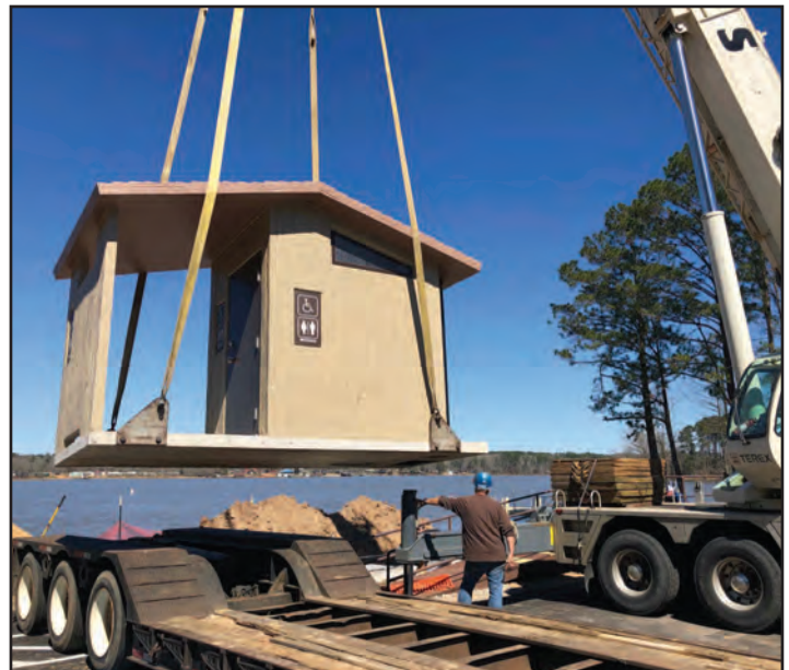
Six Mile Restroom Installation
