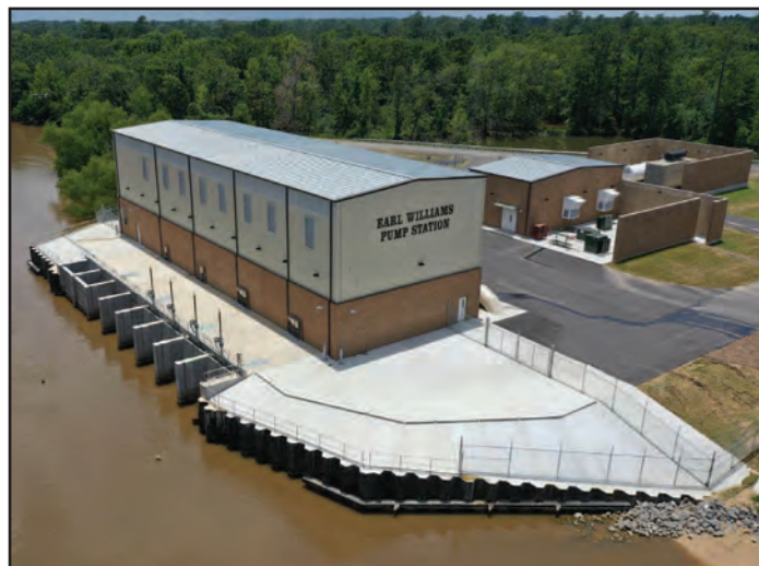
Earl Williams Pump Station
