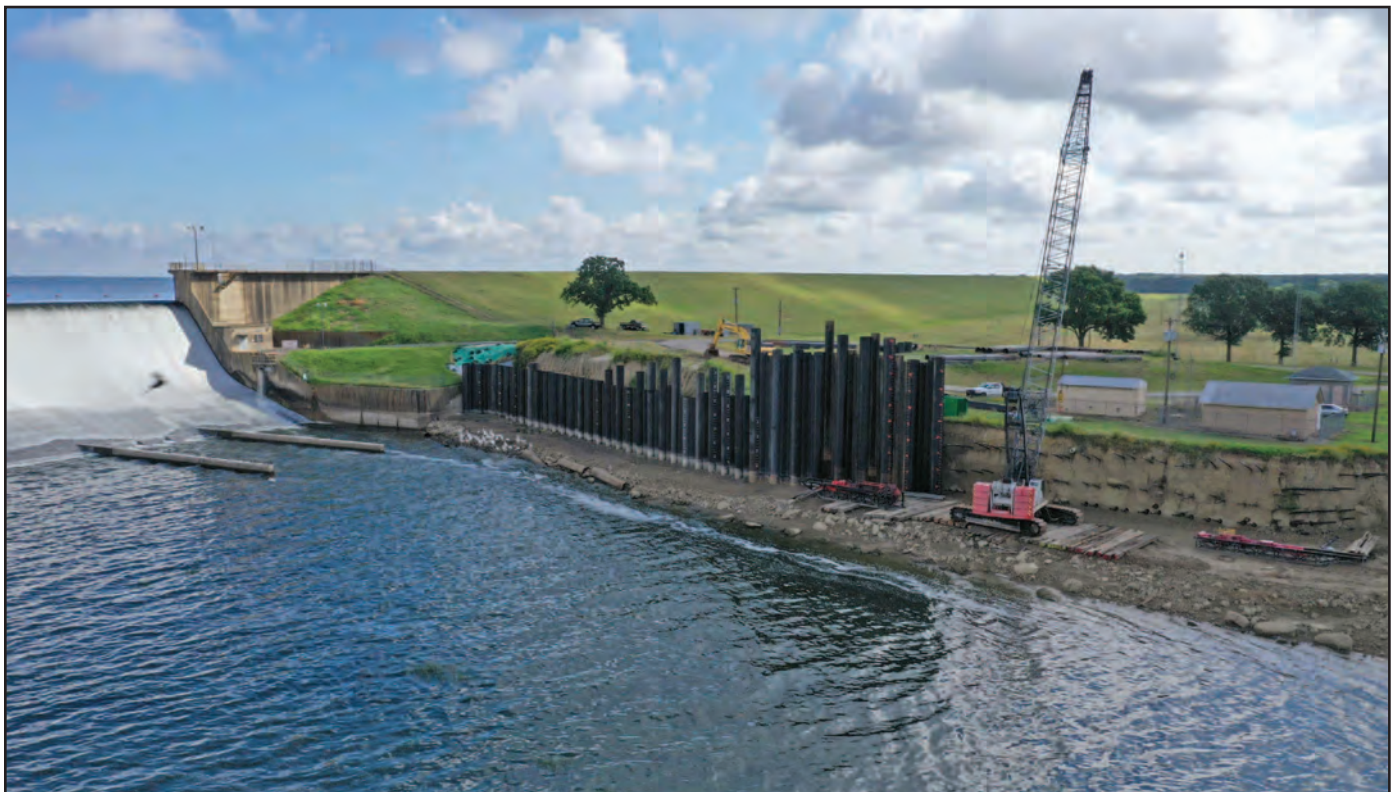
Channel Bank Stabilization Project
