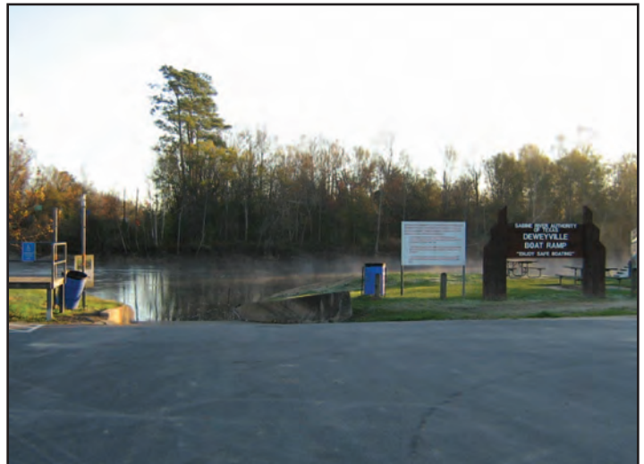
State Highway 12 Boat Ramp in Deweyville
