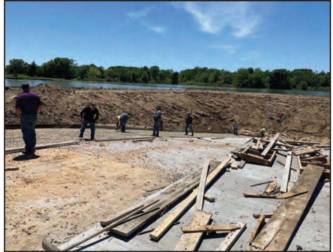
Construction of New Boat Ramp at Lake Tawakoni Recreation Site
