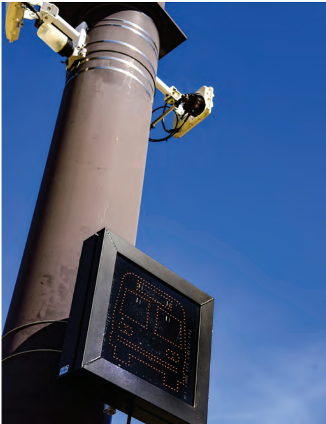
Enhancements to the signaling at the test intersection include visual and audio warnings for pedestrians and bicyclists that let them know a bus is turning.
