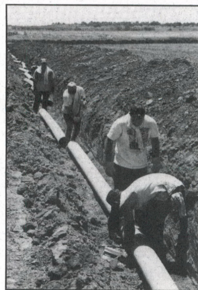
Volunteers lay the 14-mile pipeline.
