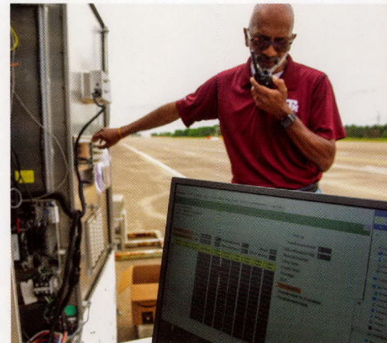
TTI's smart intersection features a variety of tools and resources for connected infrastructure and traffic signal research.
