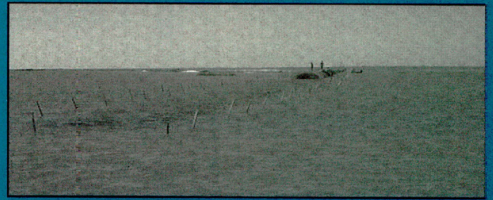
Figure 1 - Geotube construction, Galveston Island SP
