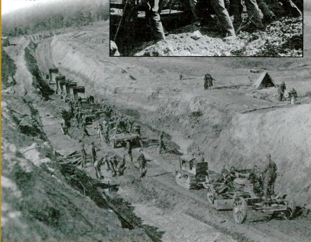
Men and machines build a dam at Daingerfield SP, ca. 1933.
