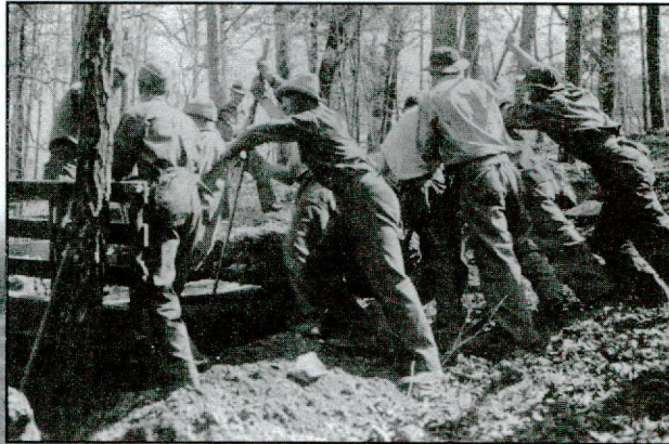
CCC Company 2891 at work on the roads.
