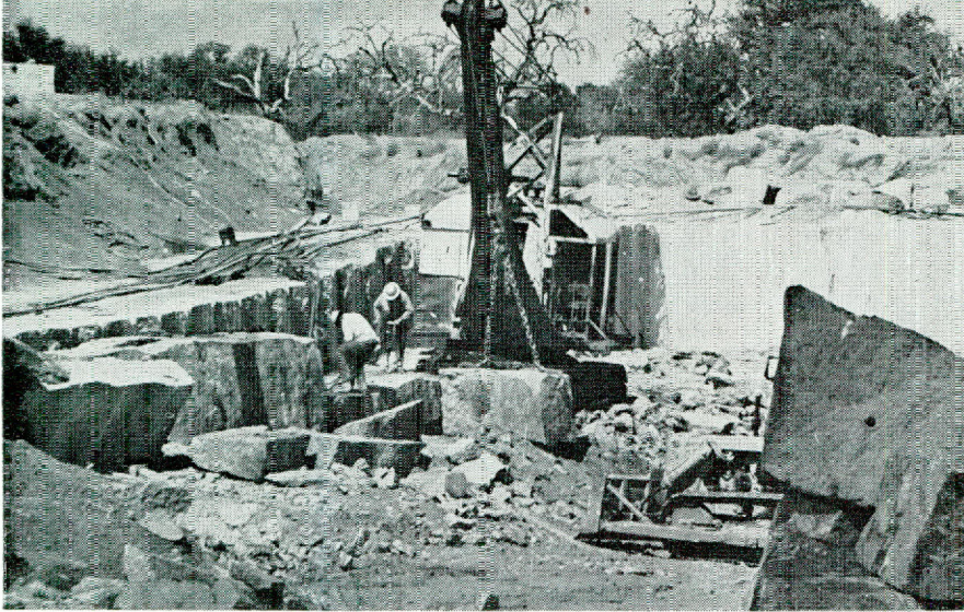
Huge boulders are blasted from the walls of this granite quarry north of Marble Falls, and loaded on gondolas for shipment to Port Mansfield. Some 300,000 tons of rock will be used on the jetties.
