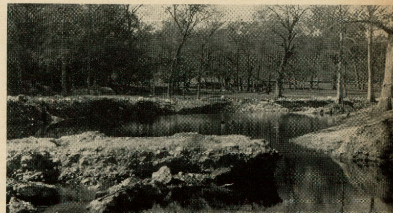
The historic September flood ravaged some of the ponds. This cut was slashed into the wall of pond Number Two.
