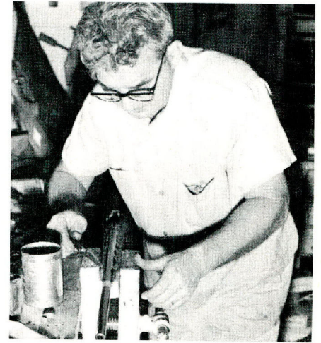
Stubby skillfully scrapes off the excess glass after it has set but just before it hardens.
