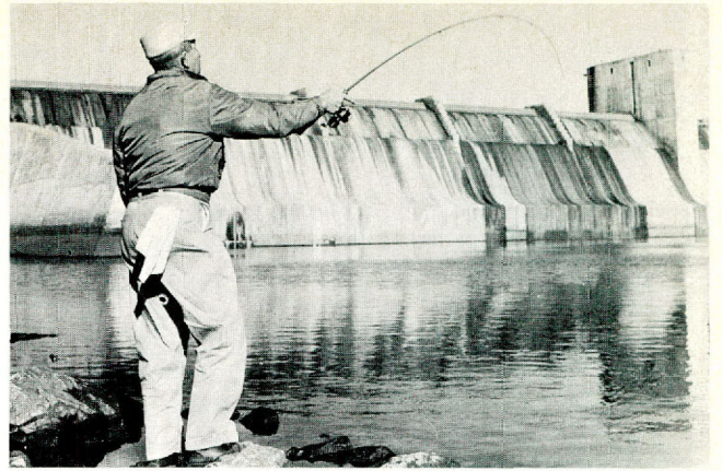
Rods bent into this success-telling arc are not uncommon below the dam gates.
