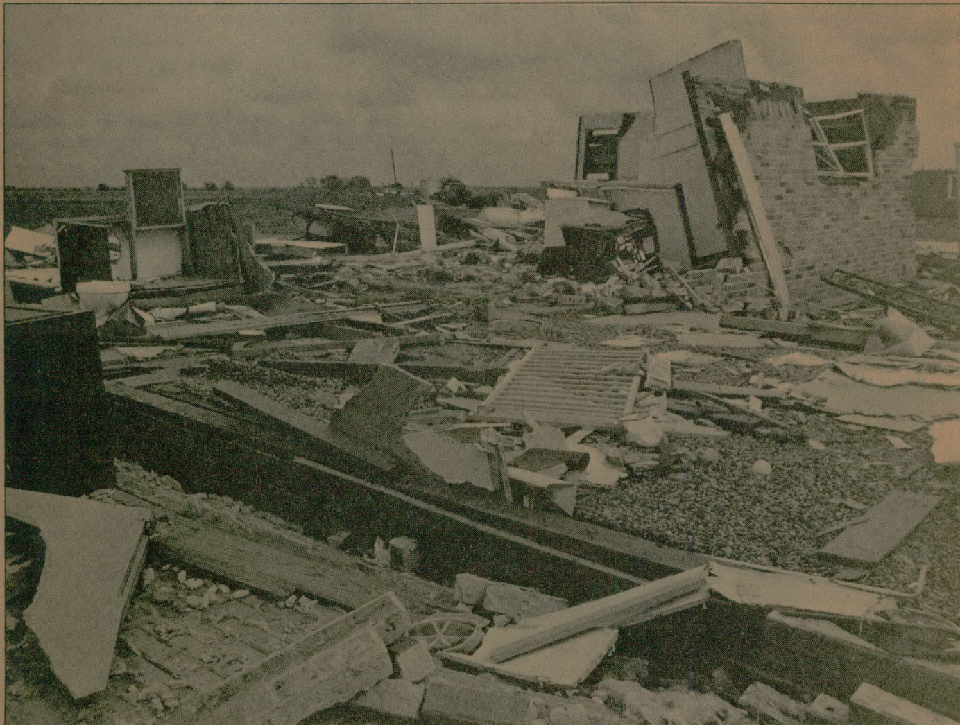
Vernon Center was spared by the tornado that struck the town April 10, but this brick home was swept almost entirely off its foundation. A section of a baby bed lies on the living room carpet. Photo by Hanaba Noack.
