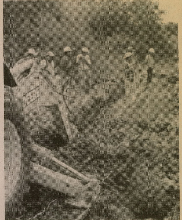
Residents of Kennedy Ridge initiated the effort to bring water and wastewater services to their community. They also provided the labor to install 14,600 linear feet of pipeline.
