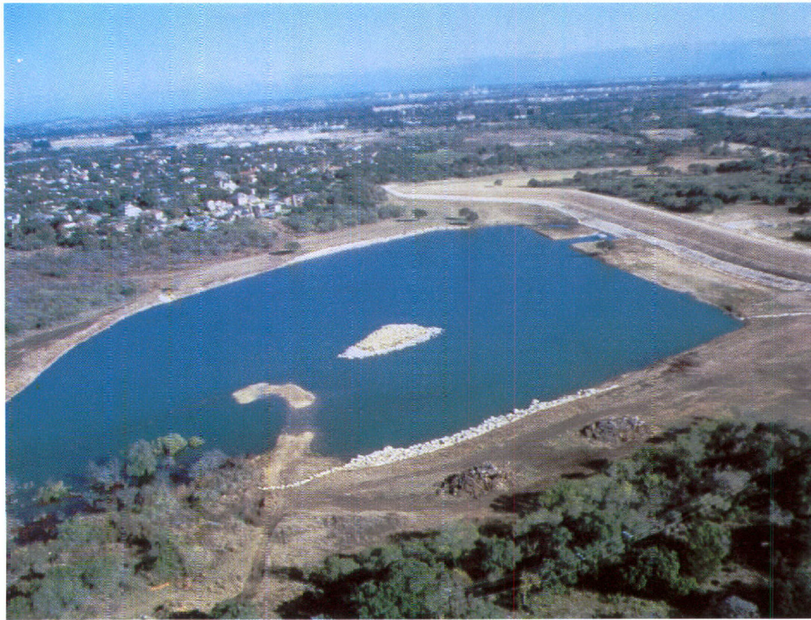
Floodwater retention dam, Salado Site 7.
