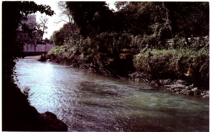
Before beautification of the SACIP flood channel in the historic King William area
