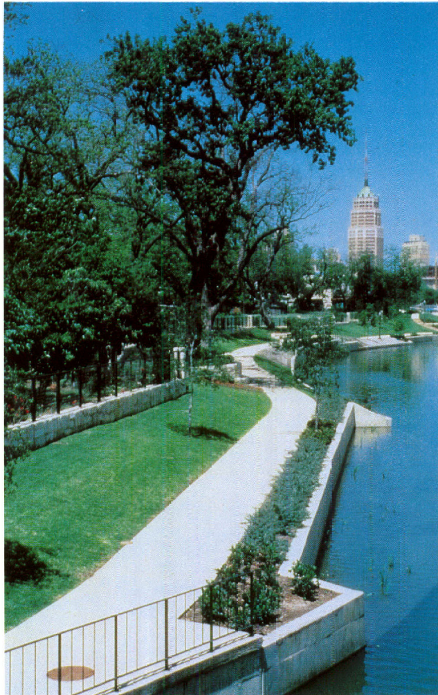
Newly completed Channel Betterments looking north from Johnson Street.
