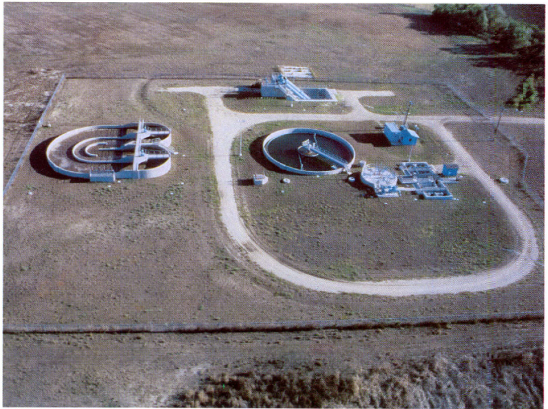
Martinez II Wastewater Treatment Plant
