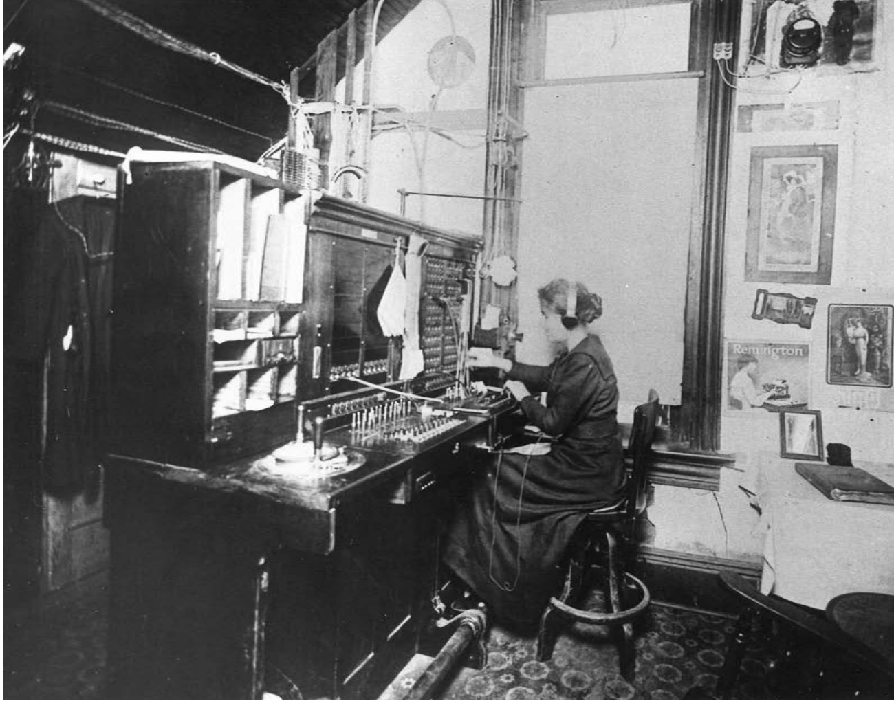
The Richardson Telephone Exchange opened in 1901. The switchboard operator worked out of a back room in Harben's Drug Store.
