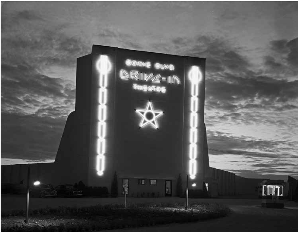
The Bowie Boulevard Drive-in was the first in Fort Worth. Like the N.W. Hi-Way Drive-in in Dallas, it was built of poured-in-place concrete with minimal decoration. Note the “Lights Out” sign at the right—it was too dark to drive in the theater unattended. The decoration was enhanced at night with neon light.
