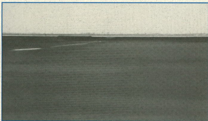
This red mud or tailings storage area is shown before the Alternative Closure Demonstration Project began. (photo courtesy of Tom Ballou)
