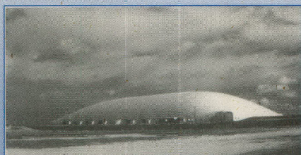
Hoechst Celanese's six-acre fabric dome keeps rainwater out of landfill and eliminates polluted runoff.
