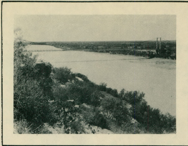
Looking downstream toward the silt sampling station which is located on the International suspension bridge between Roma, Texas and San Pedro, Mexico. The river discharge was approximately 12,000 acre feet per day and silt load 18 acre feet.
