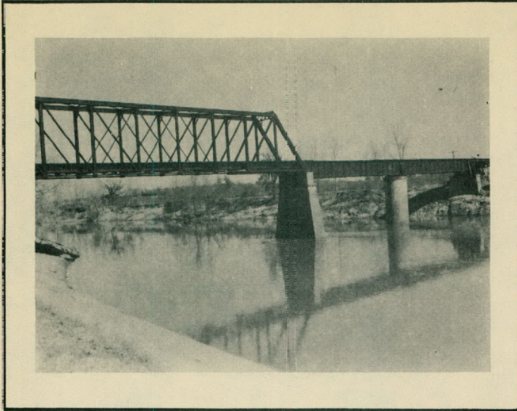
Gulf, Colorado and Santa Fe Railroad bridge at Romayor that was used for a number of years as a silt sampling station. Looking upstream. The river discharge was 11,300 acre feet of water for day and the silt load 11.7 acre feet.
