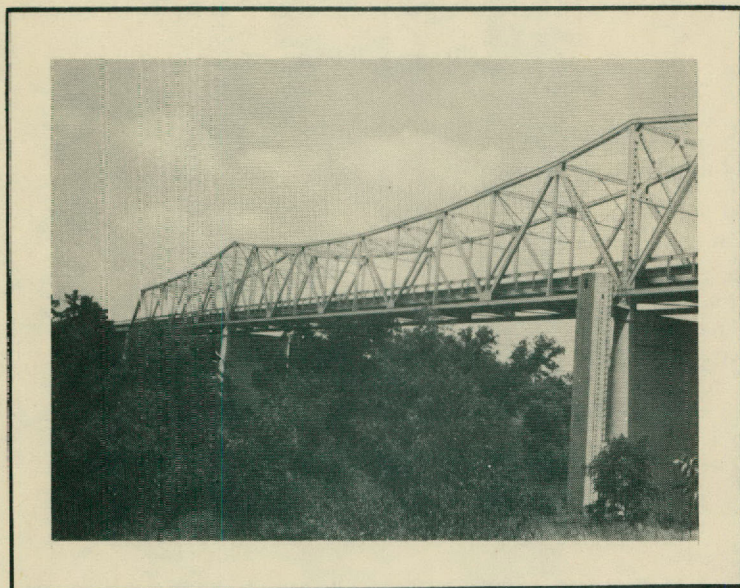
Bridge on U.S. Highway 190 that has been used since May, 1940 as a silt sampling station. It is located between Lometa and San Saba. Picture taken from downstream side of bridge.
