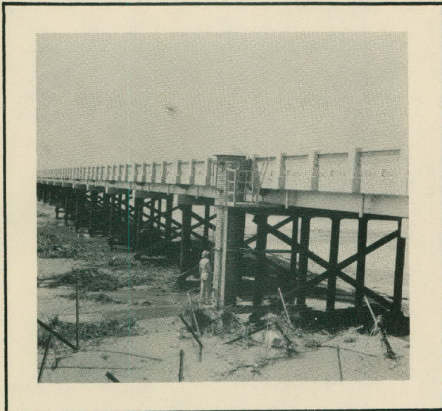
The silt sampling station is located at a bridge on State Highway 283 between Crowell and Quanah and wherever the stream channel happens to be at time water samples are obtained. The stream channel is very wide and shallow and shifts with every little rise of water from one bank to the other. At time picture was taken the USGS gaging station was "high and dry" and on the opposite bank of the stream channel.
