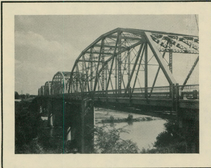
The silt sampling station at Montopolis Bridge on US Highway 183 in the southeastern edge of Austin, about 6 miles downstream from Lake Austin. Most of the water samples are obtained from second section of bridge. Occasionally, some dirty water from gravel washing plants upstream have entered the main stream channel. The original station was established at Congress Street Bridge but the gravel plant operations and reconstruction of Austin Dam caused its removal further downstream to the Montopolis Bridge site.
