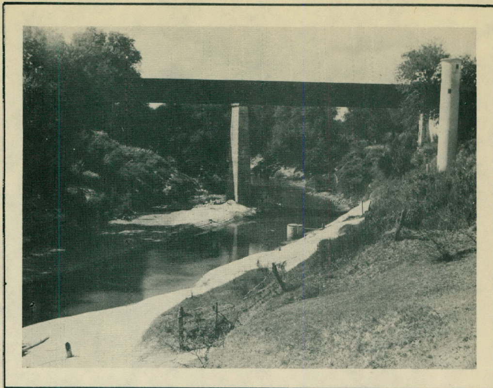
San Antonio, Uvalde and Gulf (Missouri Pacific) Railroad bridge used as a silt sampling station. This station, or at a small concrete dam one-foot high and about 150 feet below it, have been used for the past 25 years as sites for collecting water samples for silt determinations. One silt sample collector, Mr. Carl Franze, has been collecting the daily water samples during the long record at this station. This station is located about 25 miles upstream from Lake Corpus Christi. The drainage area between this station and the Lake is approximately 1,000 square miles.
