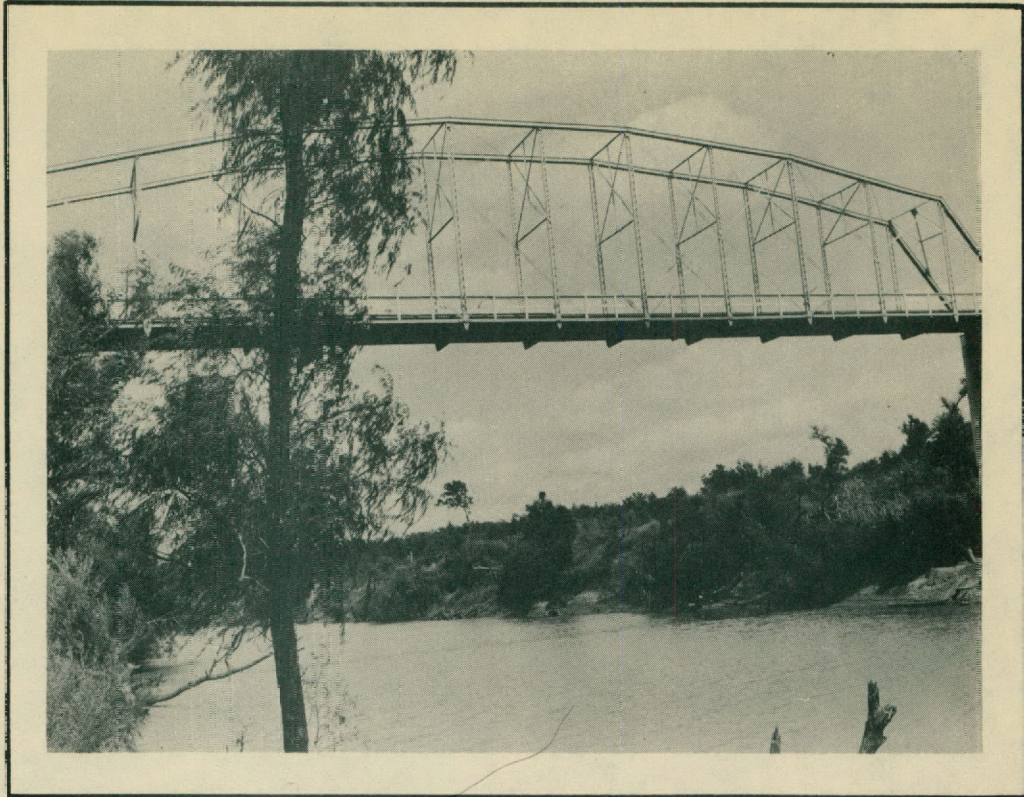
Old Red Eluff Bridge used as silt sampling station prior to May 24, 1940. During World War II it was blown up by Corps of Engineers for the steel. A new bridge was constructed about \frac{1}{2} mile above and it is now used as a silt sampling station. Looking upstream.
