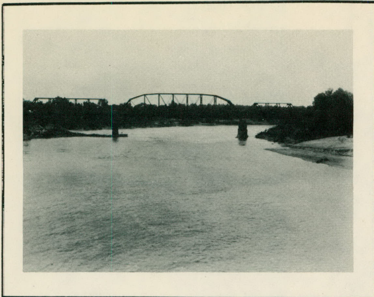
Looking upstream from silt sampling station.
