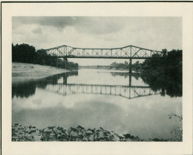
Silt sampling station at bridge on US-Highway 50 in Richmond. Looking downstream. During the past 28 years, 919,031,170 tons or 602,027 acre feet of silt have passed this station into the Gulf of Mexico. This amount is sufficient to have jeopardized the economic life of a lake similar to Possum Kingdom Dam on the same watershed (capacity 750,000 acre feet). The river discharge during the 28 years amounted to 152,240,180 acre feet. Prior to 1932 the silt station was located at a bridge near Rosenberg.
