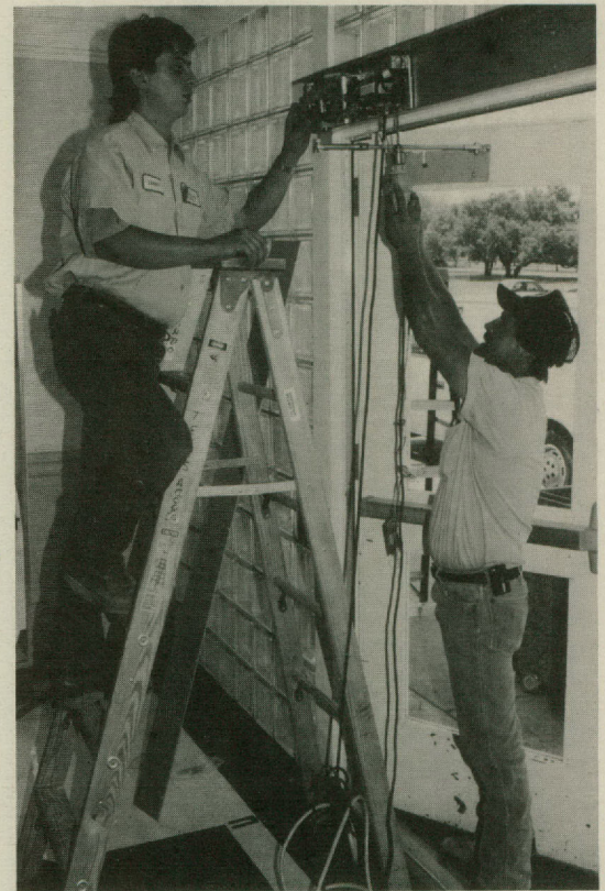
Installation of electric door openers makes Lee College accessible to everyone
