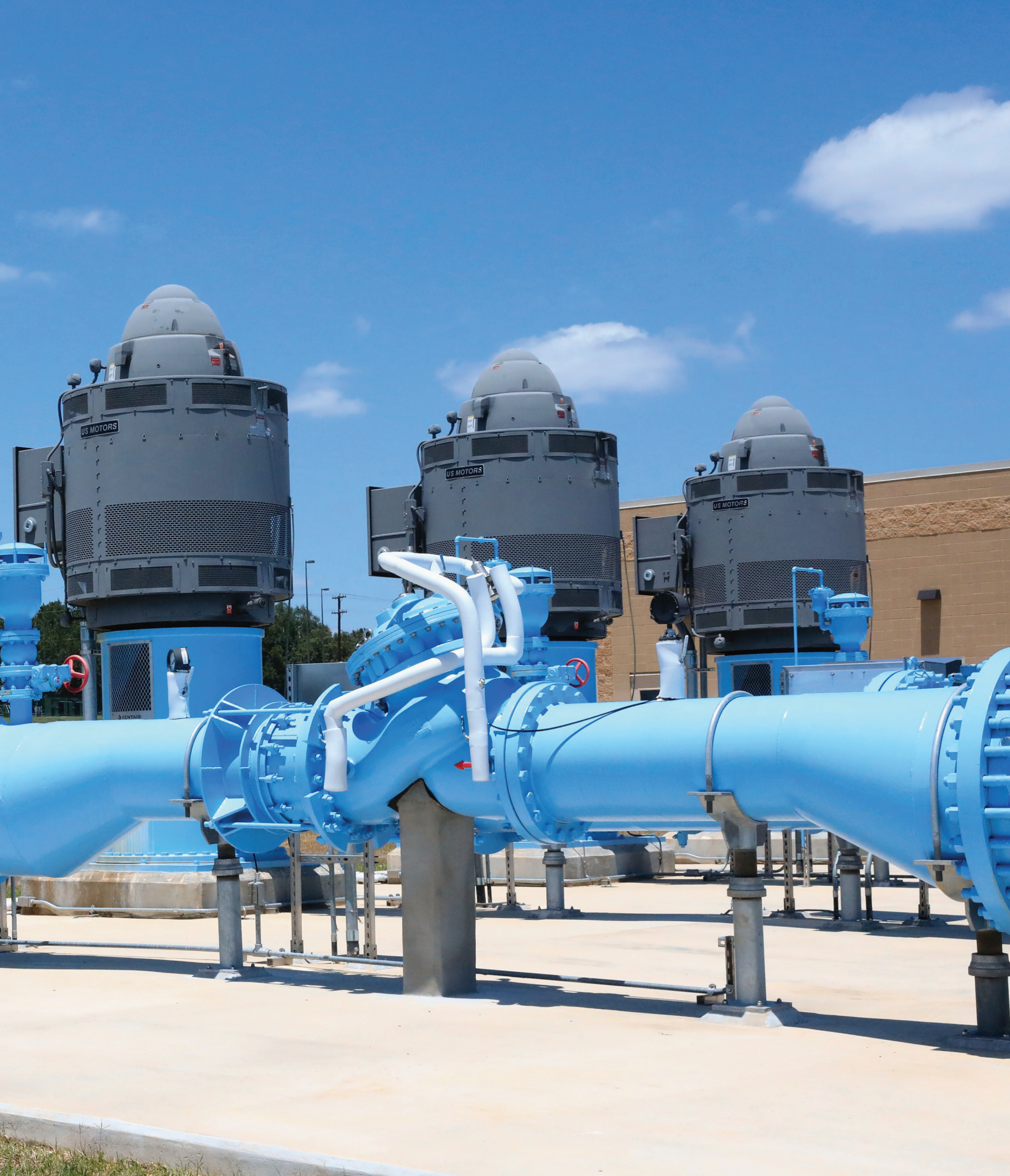
HIGH SERVICE PUMPS AT THE AQUIFER STORAGE & RECOVERY FACILITY [ASR] IN SOUTH BEXAR COUNTY
