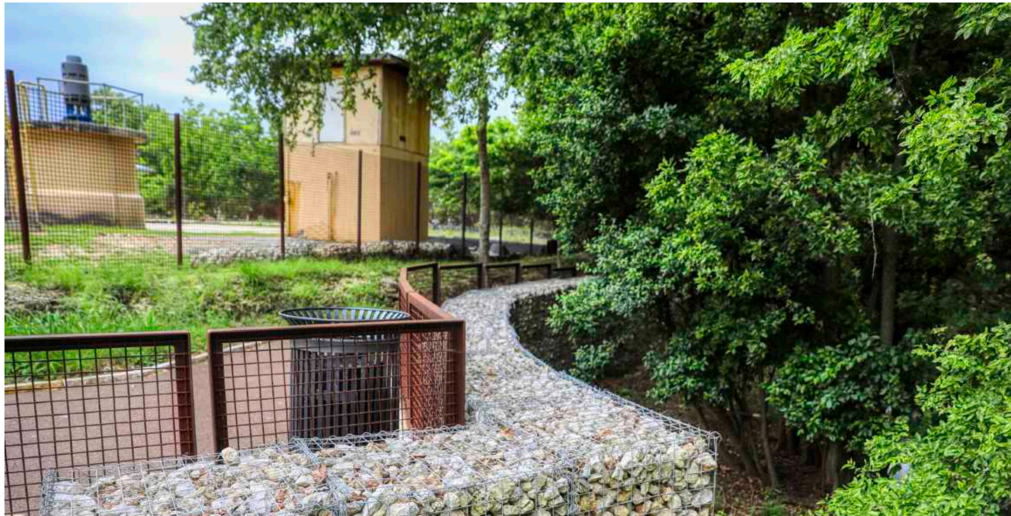
Gabion wall protecting the spring openings along the Comal.
