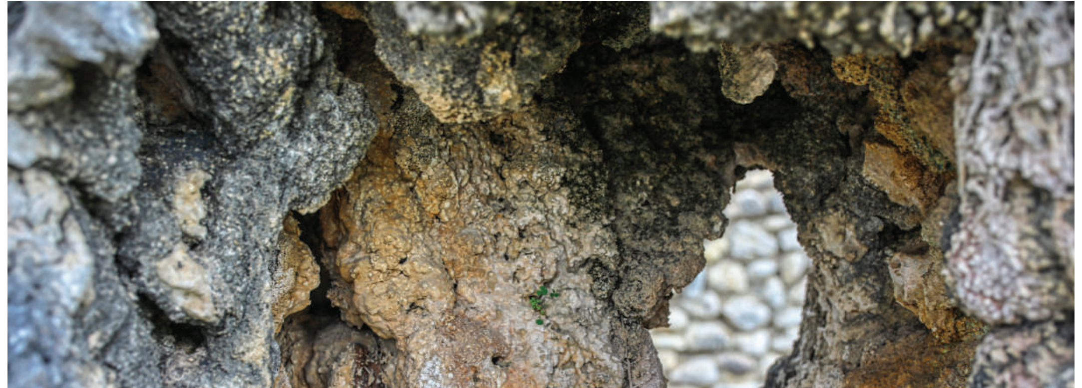
Old Stone Fountain Well at the Headwaters of the Comal.
