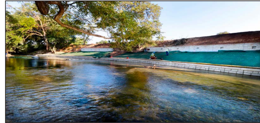
Photo: Bank Stabilization.
