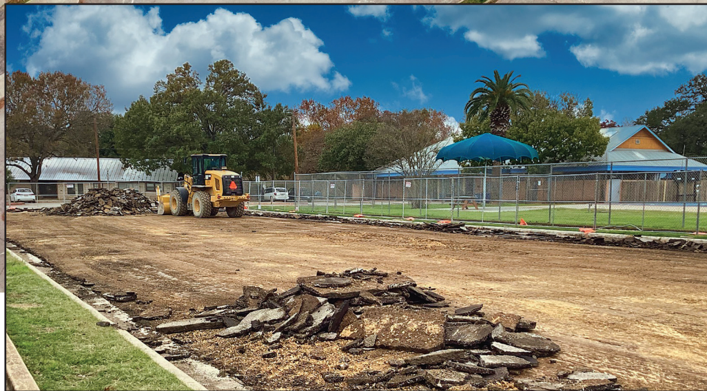
Clearing parking lot for construction.
