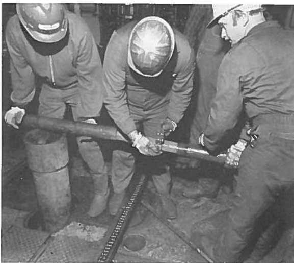
Helicopters (top) are used to ferry crew changes to the drillship, JOIDES Resolution. Scientists test new ocean drilling equipment (above, right), while staff members retrieve a 30-foot core from the drillship's core barrel (above, left).
