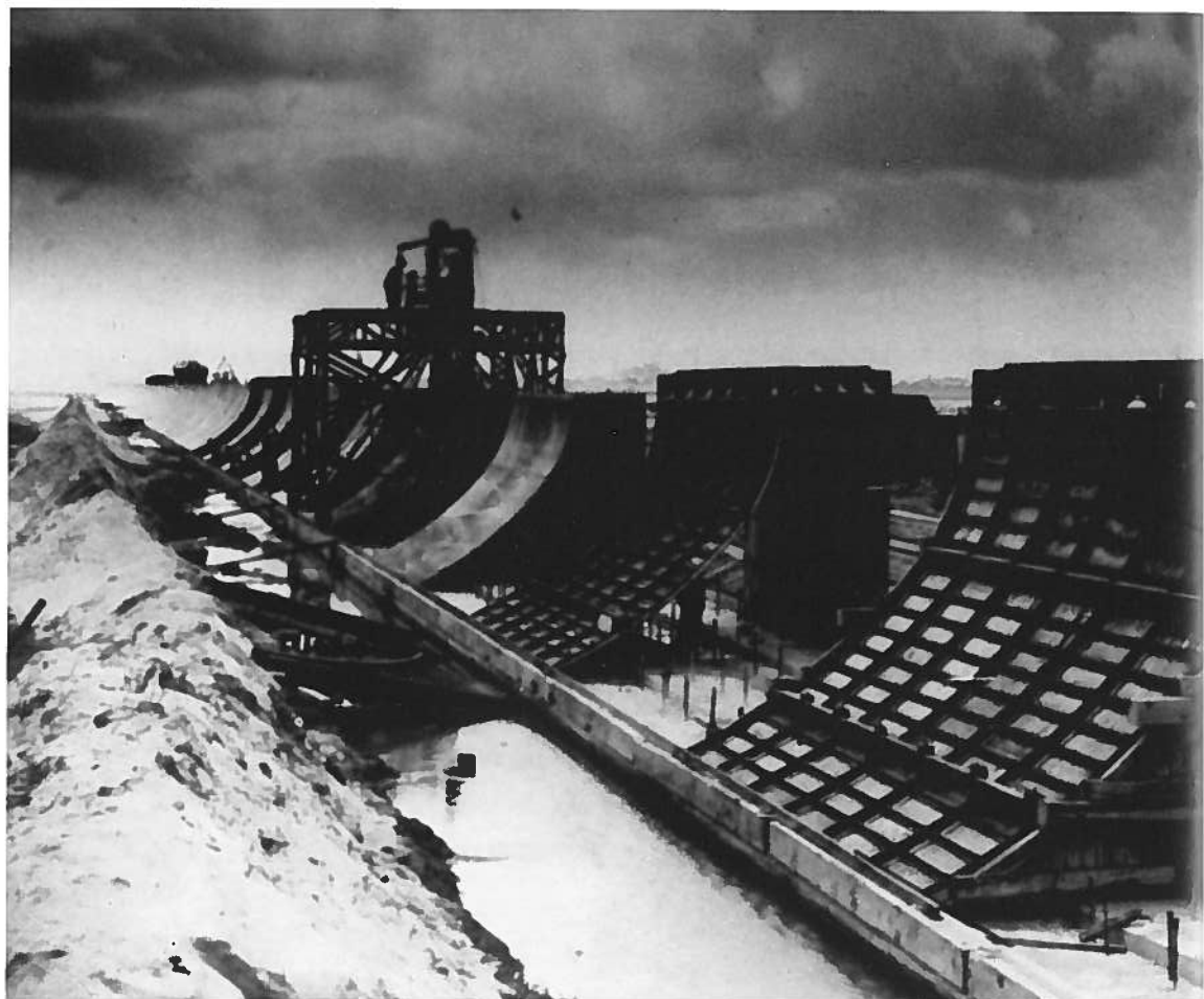
Galveston's 17-foot-high, 10-mile-long wall was completed over a period of 61 years. When the wall went in place there was a veritable sea of sand in front of the barrier.
