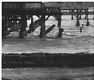
Galveston's groins went into place in 1936. They help protect the seawall from erosion.
